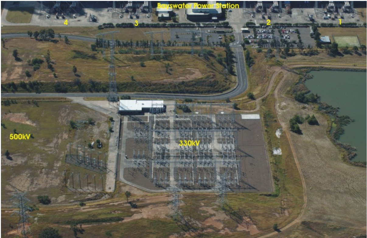
Bayswater 330kV Switchyard and Bayswater Power Station showing units 1 to 4 generator transformers.
