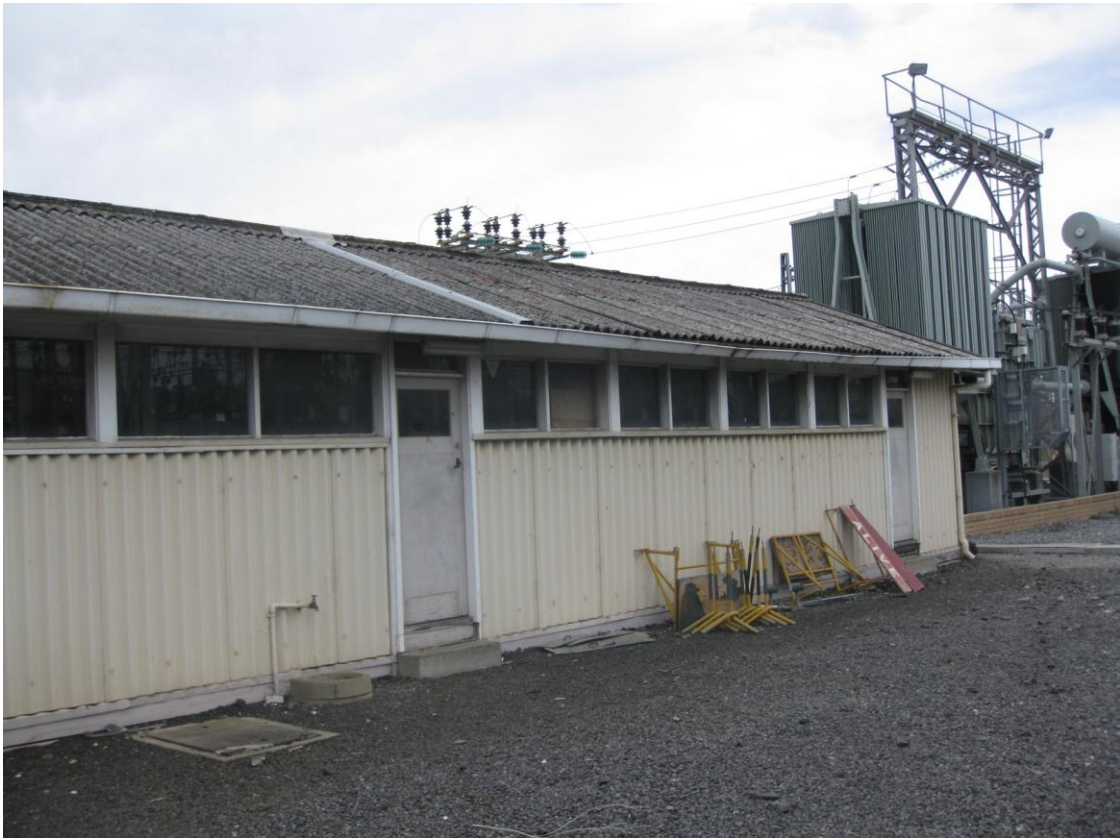
Photo No.1 – Control Room Building – Typical exterior (South side of building).
