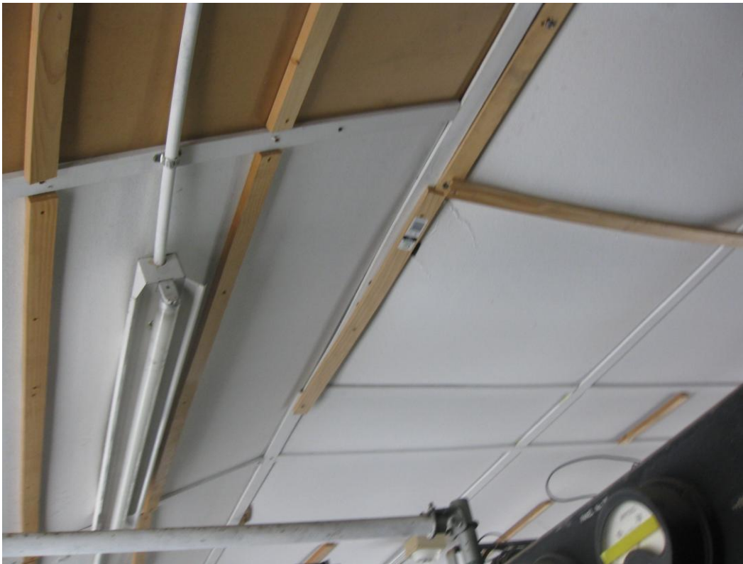
Photo No.5 – Control Room Building – Typical “Canite” ceiling.
