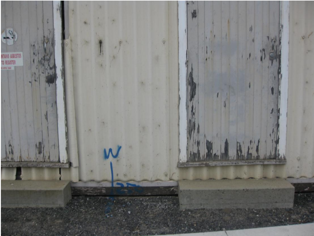
Photo No.7 – Control Room Building – T & G Timber doors (North wall)
