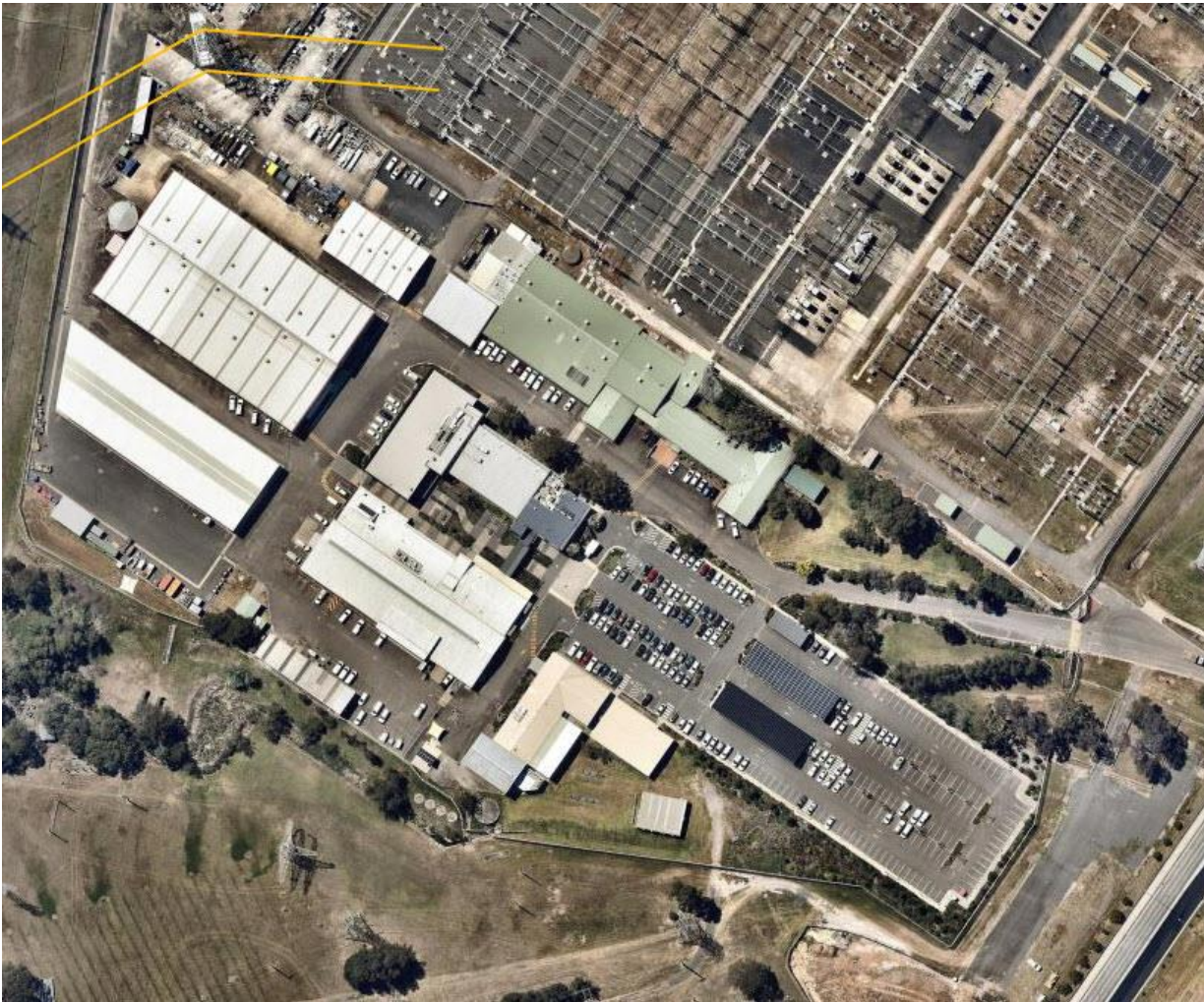
Aerial of Metropolitan Area Centre
