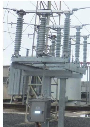
Typical disconnector installation
