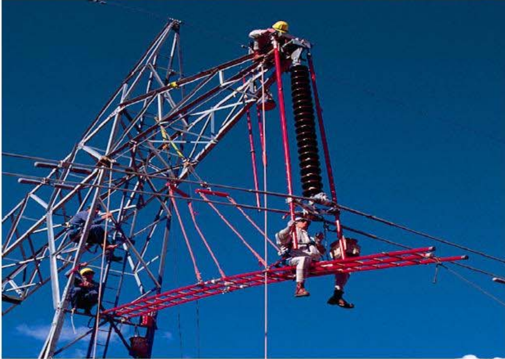
Bare-hand live line maintenance in the Tamworth area
