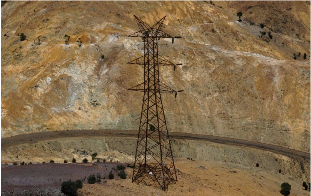
Figure 3: Steel lattice tower (weather resistant steel)
