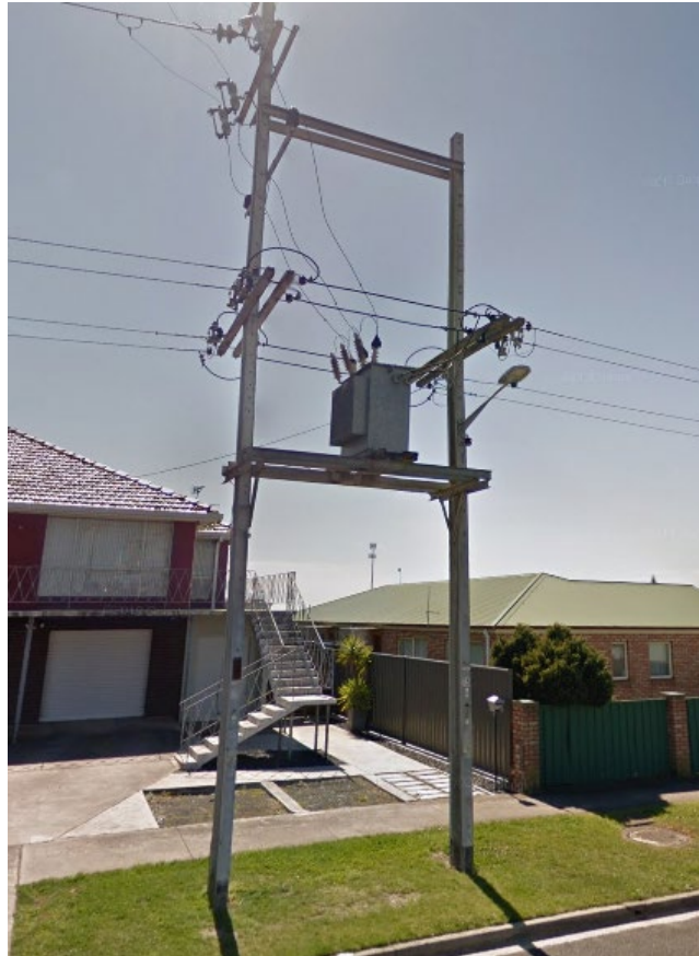
Figure 5: Transformer H-structure
