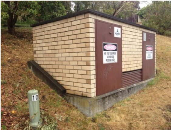
Figure 1 Block wall kiosk (1977)
