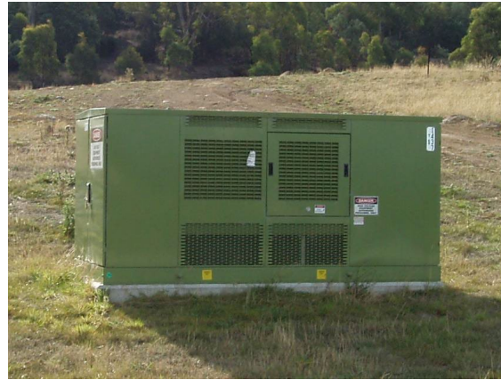
Figure 2 Modern steel kiosk (2012)
