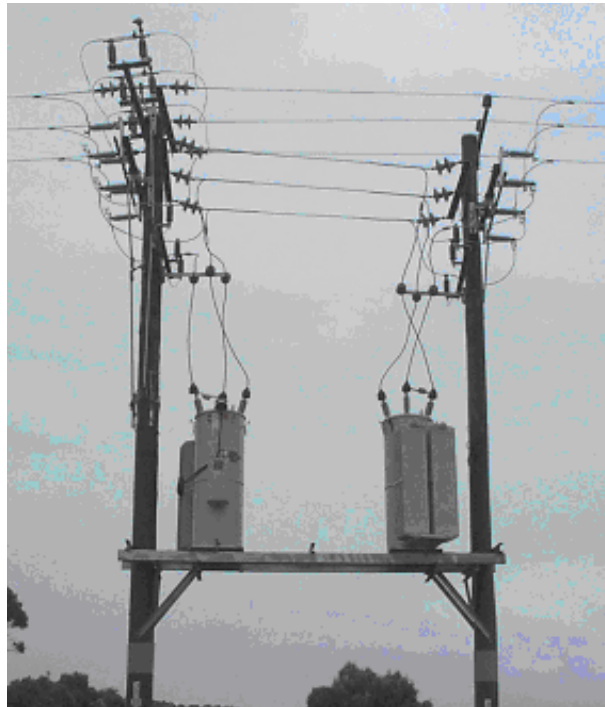
Figure 6: Typical three phase HV regulator site
