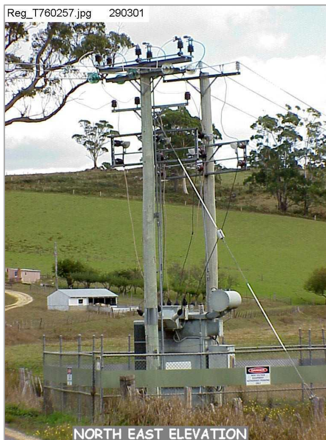
Figure 6: Typical three phase HV regulator site
