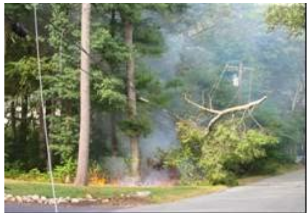
Photo 4: Multiple broken conductors on distribution network
