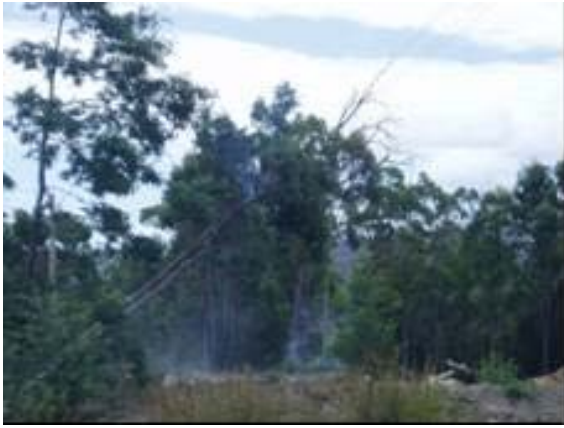
Photo 1: High voltage distribution conductor clash
