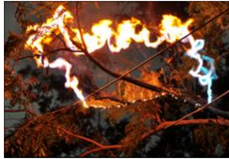
Photo 2: Phase-to-phase fault
