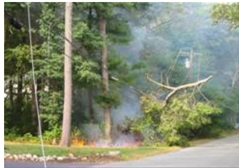
Photo 4: Multiple broken conductors
