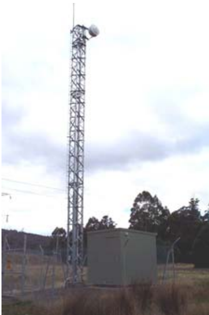
Figure 11 - An example of a steel lattice monopole support structure
