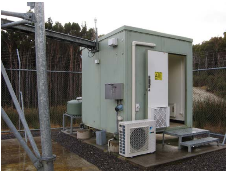
Figure 19 - An example of a transportable steel clad polystyrene telecommunications hut
