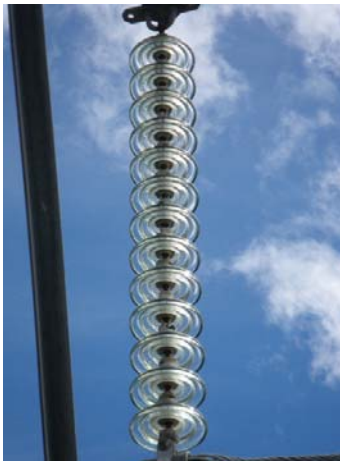
Figure 1: 220 kV glass disc insulator assembly
