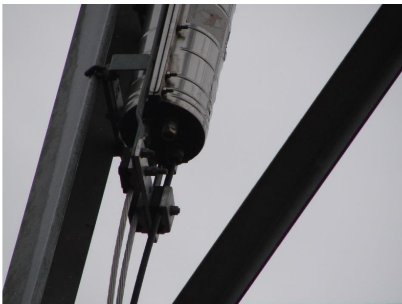
Figure 15: OPGW Splice Pod
