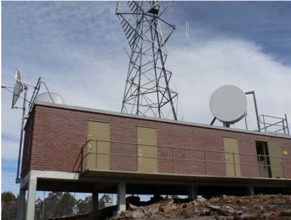
Figure 20 - An example of a brick/masonry telecommunications building
