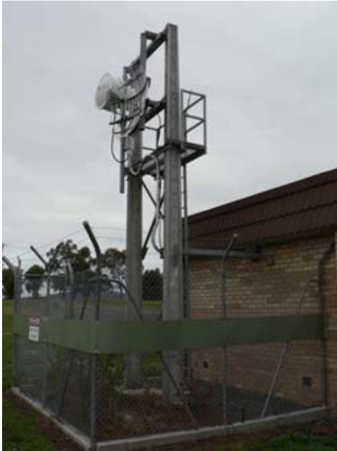
Figure 14 - An example of a twin concrete stobie pole support structure
