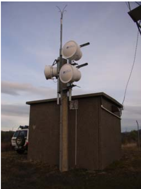
Figure 13 - An example of a single concrete stobie pole support structure
