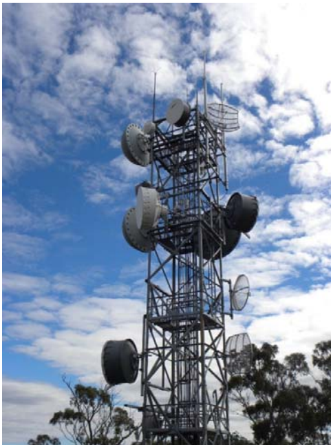
Figure 10 - An example of a steel lattice telecommunications tower
