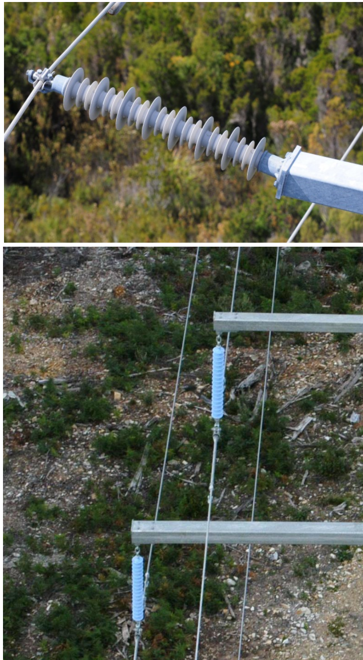
Figure 5: Post and long rod synthetic insulators
