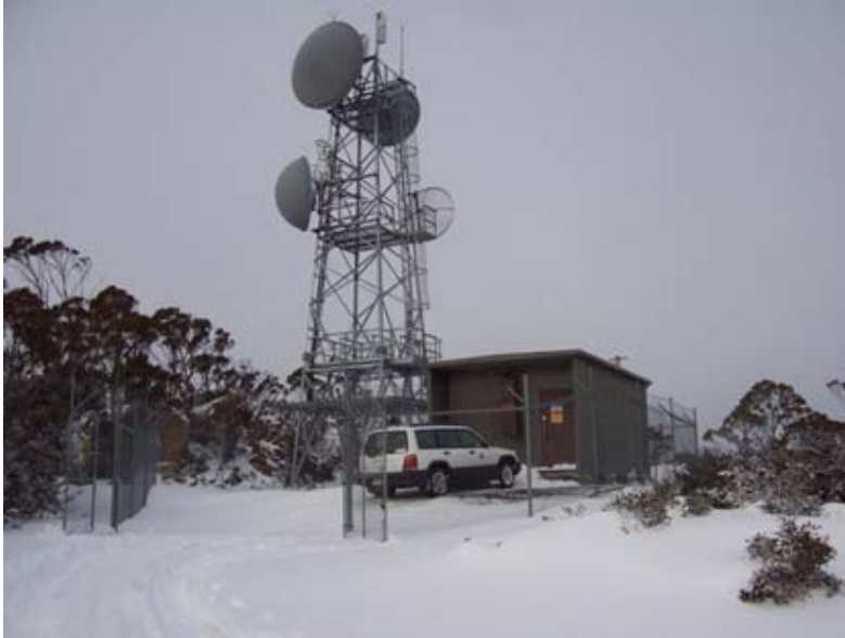
Figure 17 - An example of a pre-fabricated concrete telecommunications hut
