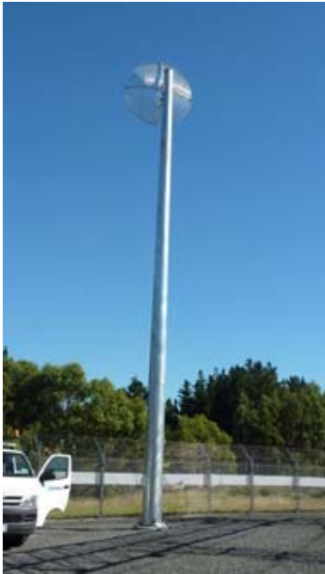
Figure 12 - An example of a tapered hollow steel monopole support structure
