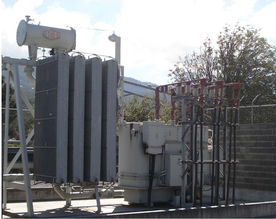
Figure 34: Tyree 10/15 MVA
