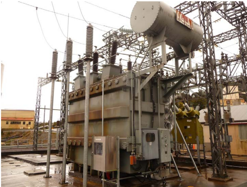
Figure 50: ABB (Tyree) 20/36 MVA RB-T2
