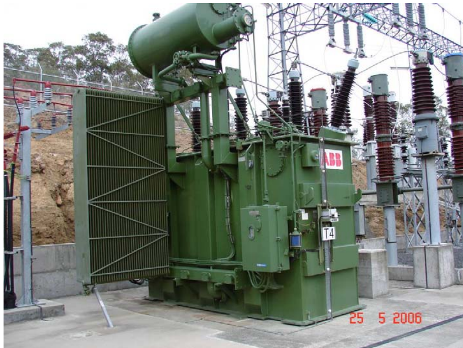
Figure 38: 25/17 MVA Meadowbank Transformer MB-T4
