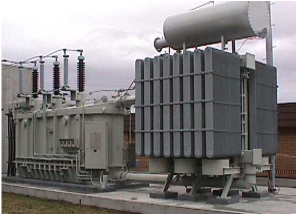
Figure 55: Stromberg 36/60 MVA
