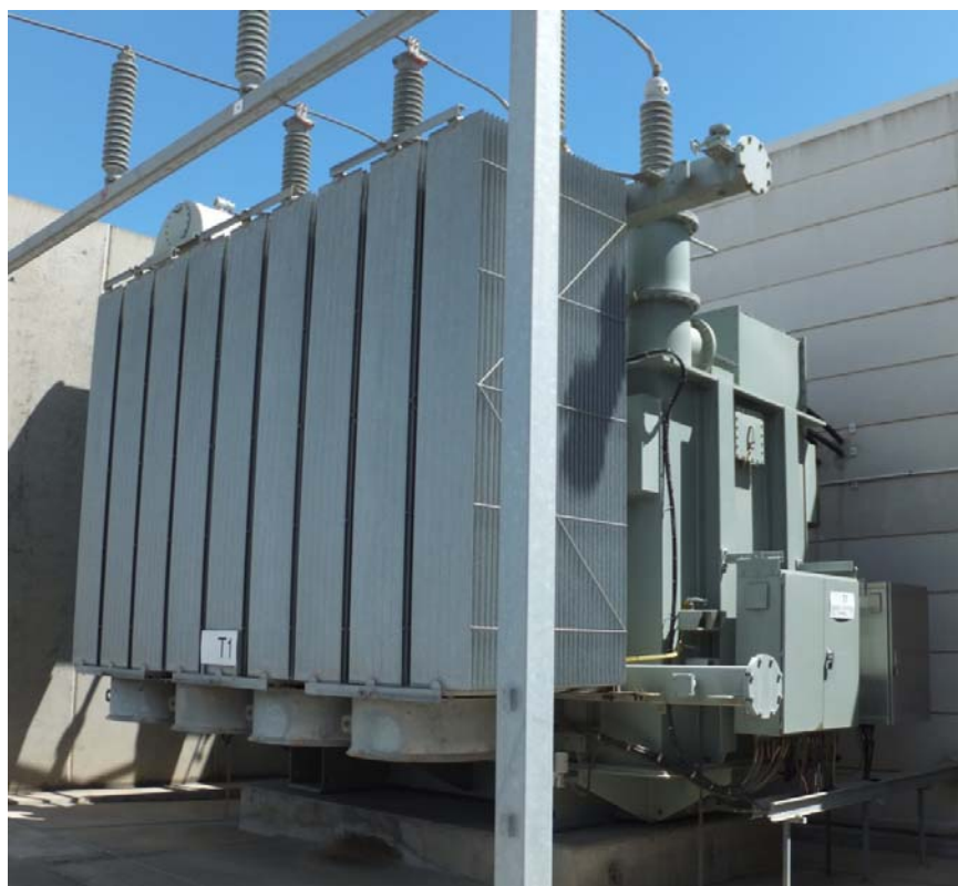
Figure 66: Alstom 65/90 MVA
