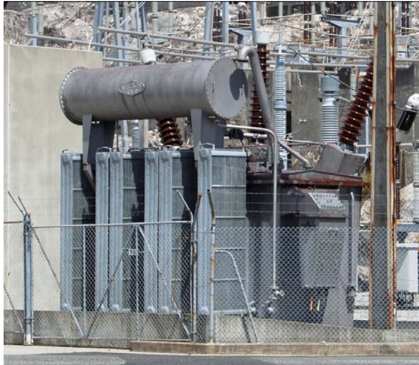
Figure 37: Wilson 10 MVA (before and after bushing replacement)
