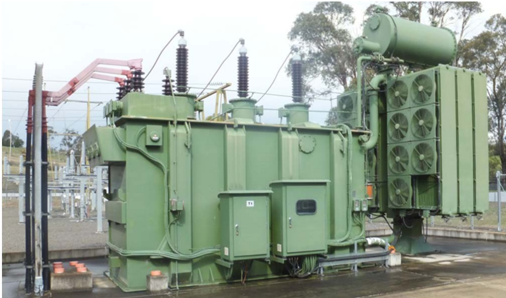
Figure 48: ABB 30/50 MVA
