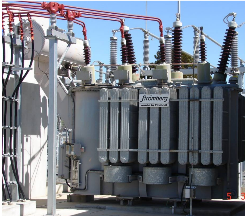
Figure 43: Stromberg 20/30 MVA
