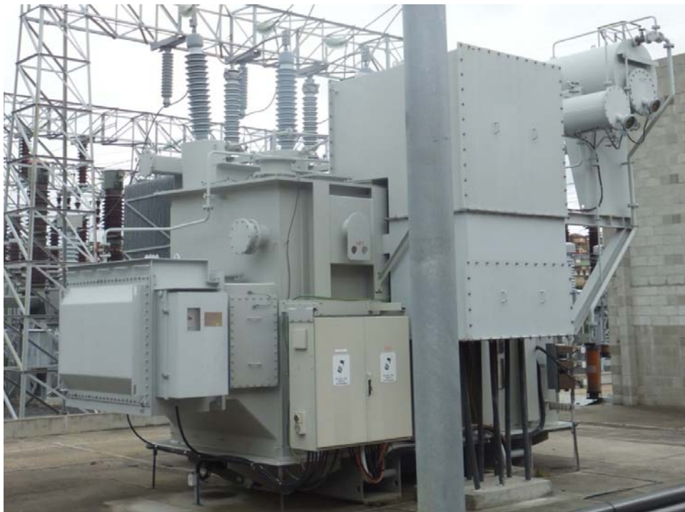
Figure 51: Alstom 30/60 MVA
