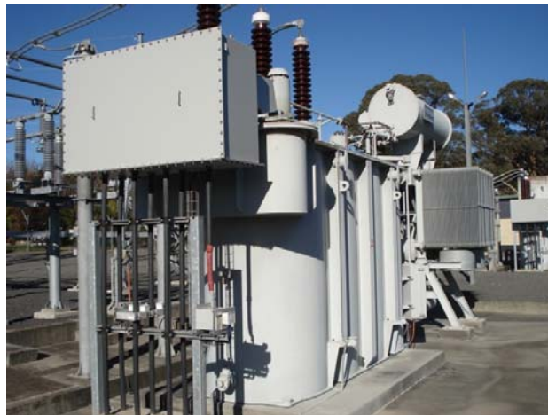
Figure 57: Stromberg 19/31.5 MVA (with new cable box)
