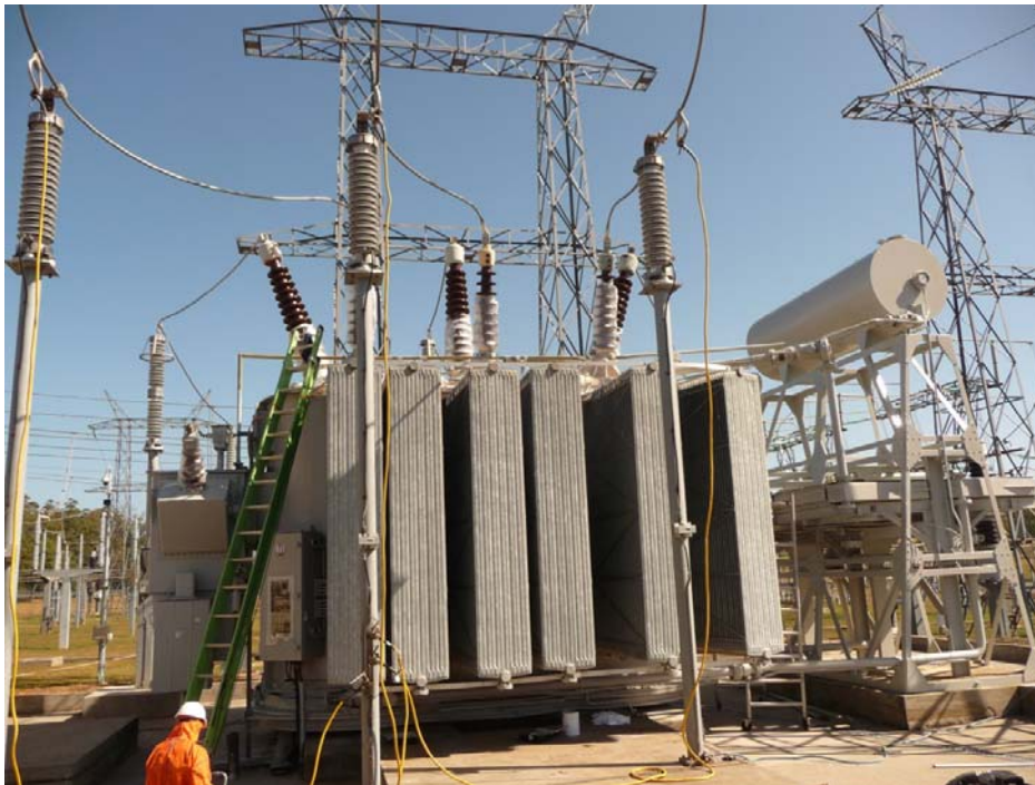
Figure 27: Network transformer T1 at Sheffield Substation
