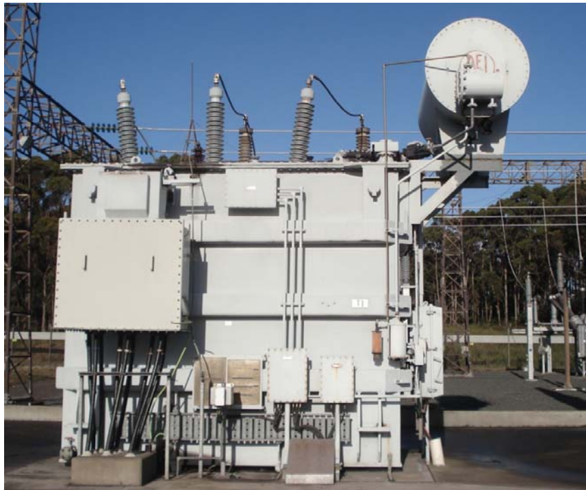
Figure 40: AEI 15/22.5 MVA
