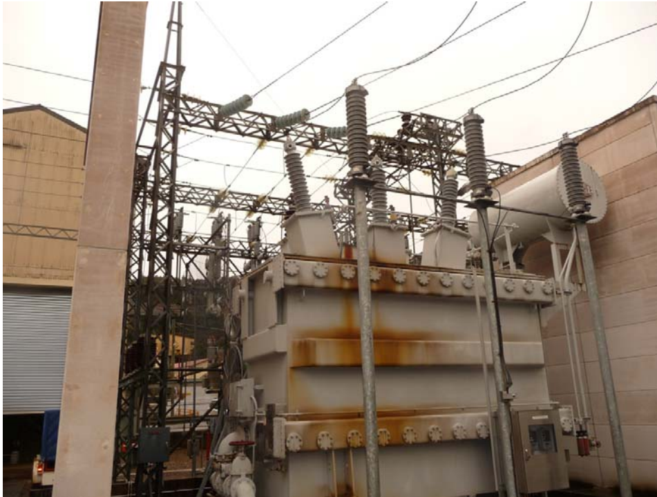
Figure 50: ABB (Tyree) 20/36 MVA RB-T2
