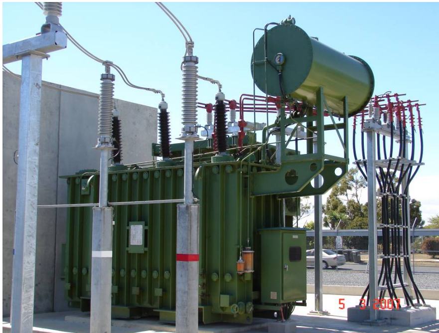
Figure 39: ABB 20/30 MVA
