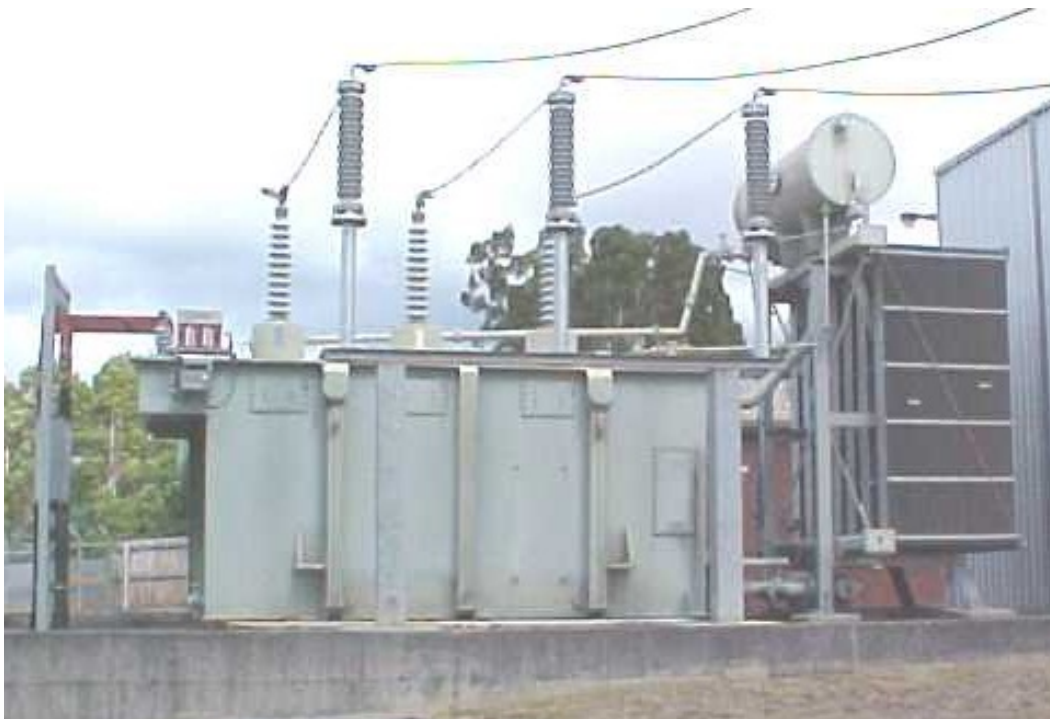
Figure 59: Tyree 30/50MVA (old photo with SRBP bushings)
