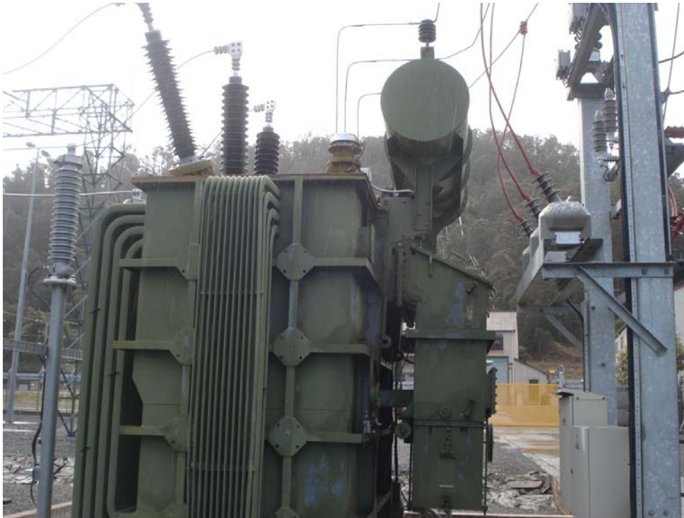
Figure 32: BGE/EPM 5 MVA (old photo having gooseneck and SRBP bushings which have been replaced)
