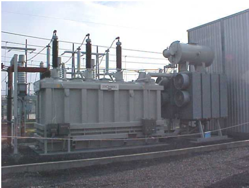
Figure 54: Stromberg 18.9/31.5 MVA
