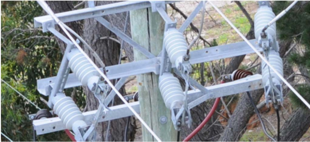
Figure 7: Typical high voltage link vertical arrangement in its closed position
