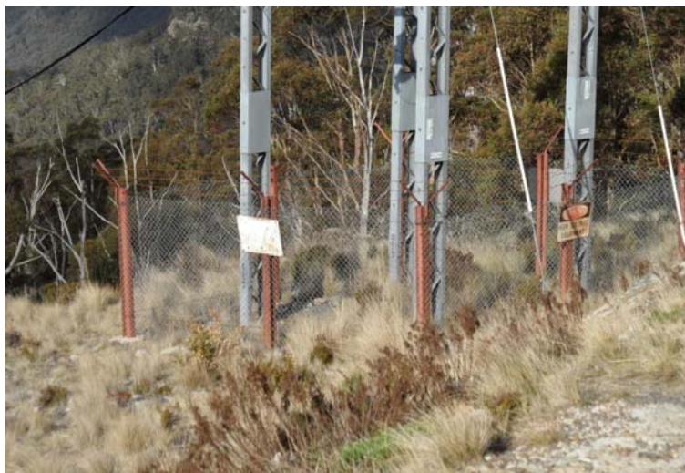
Figure 34: Anti-climbing Barrier with Faded Signage
