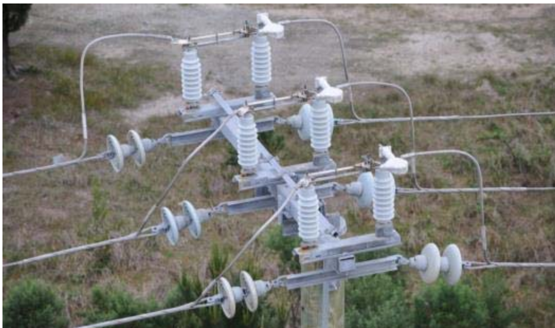
Figure 6: Horizontally operated air break switch
