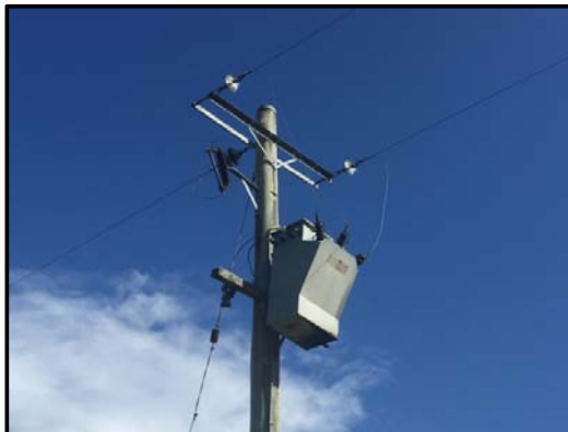
Figure 2: A SWER isolating transformer with 6/20 EDO SWER fuselink
