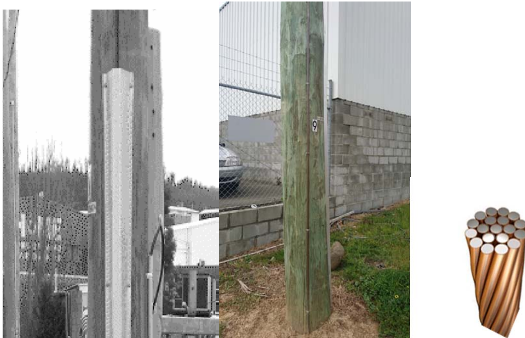
Figure 16: Pole copper earthing conductor with steel security guard to drawing D-OH1-1.8/30 and the new alternative copper clad steel rod kit used now in repeat theft locations.
