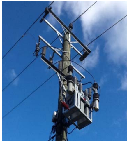
Figure 9: Pole mounted ABB capacitor bank
