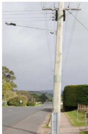
Figure 28: Staked wood pole with possum guard
