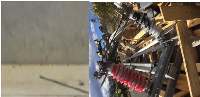
Figure 14: examples of cut- safe secured cracked insulators replaced in 2015/16.
