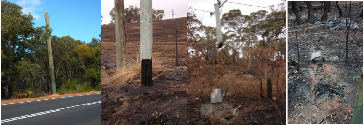
Figure 10: An intumescent coated wood pole and poles lost to reduce risk of CCA afterburn
