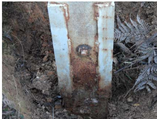
Figure 20: Poor condition steel and concrete (Stobie) pole
