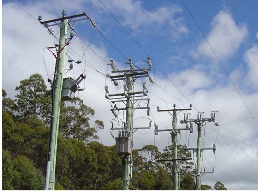
Figure 9: Pole mounted 22 kV switchgear at Derwent Bridge Substation
