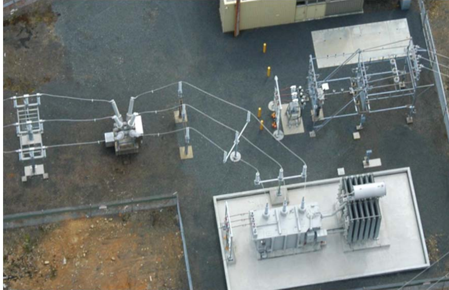
Figure 10: 22 kV switchgear at Que Substation
