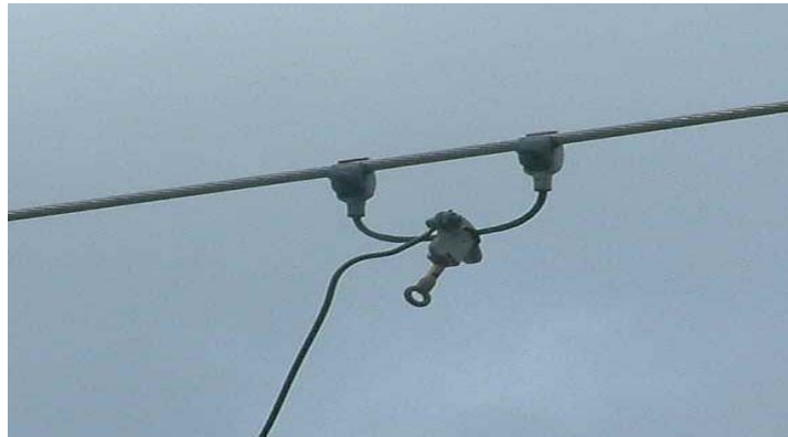
Figure 10: Live line clamp connected via D-clamp
