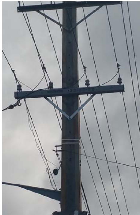
Figure 6: Fibreglass (FRP) LV cross arm in trial
