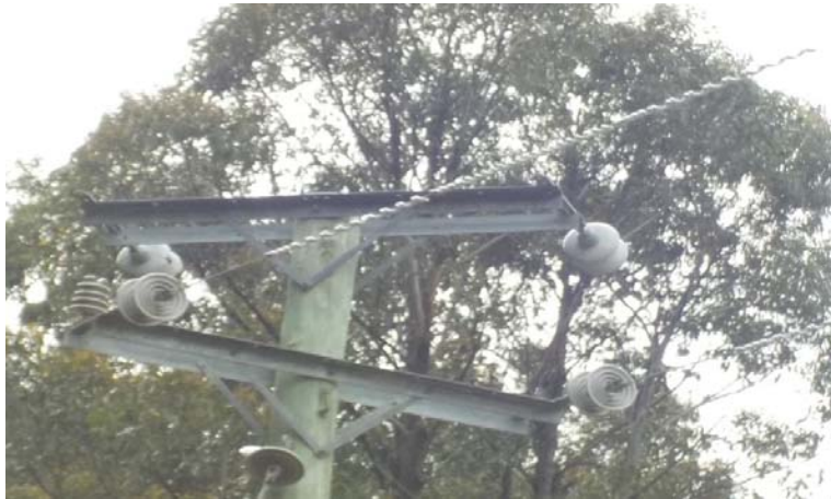
Figure 11: Three in series HV spiral dampers per conductor on a long span
