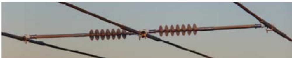
Figure 30 shows a HV mid span spacer set for AAC damping galloping solution
