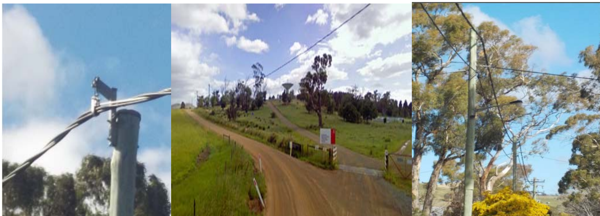
Figure 32 existing non-metallic screened (NMS) HV ABC conductor
