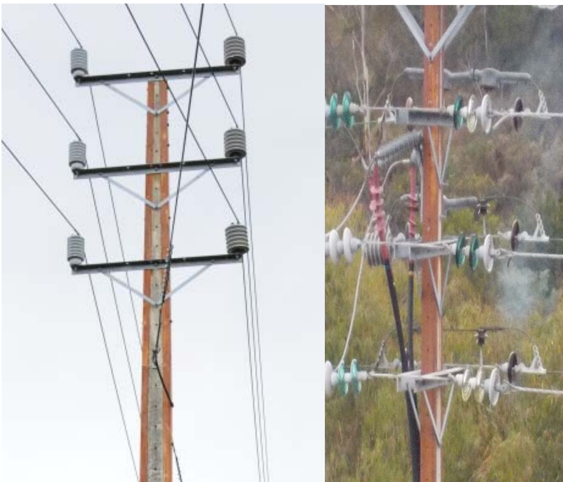
Figure 4: Steel HV cross arms and insulators on dual circuit 33kV and 33 kV and 11kV circuits on a stobie pole
