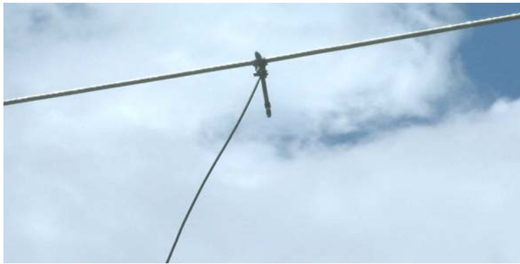
Figure 9: Live line clamp directly connected
