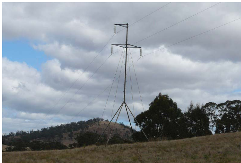
Figure 10: Kay pole installed on Triabunna Spur transmission line
