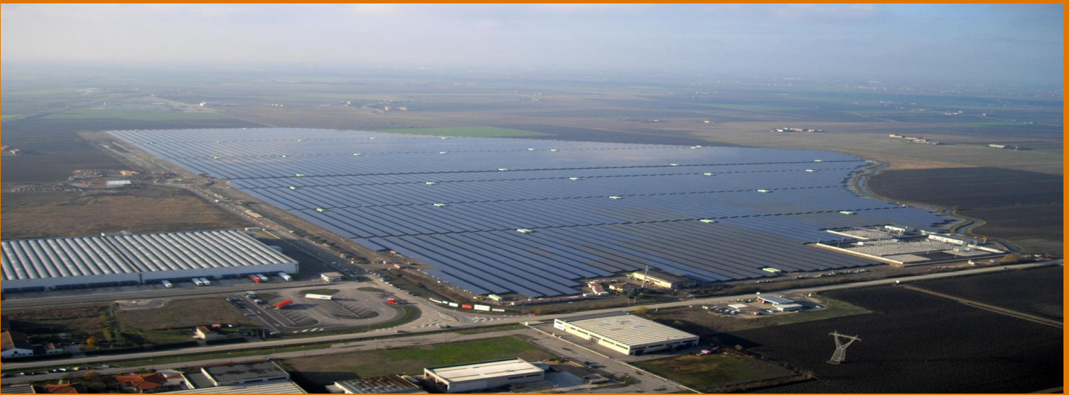
SunEdison's 70 MW power plant at Rovigo, Italy
