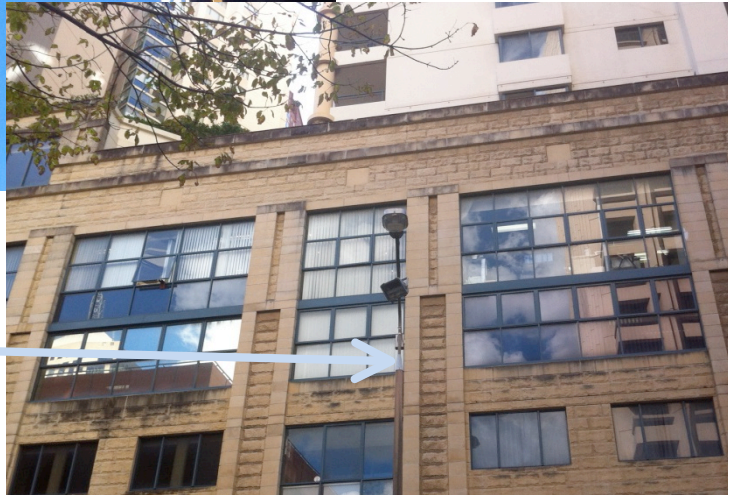
Ausgrid 'Lighting Solutions' security floodlighting for third-party customers on dedicated street lighting poles
