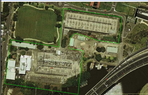
Aerial view of Richmond Terminal Station
