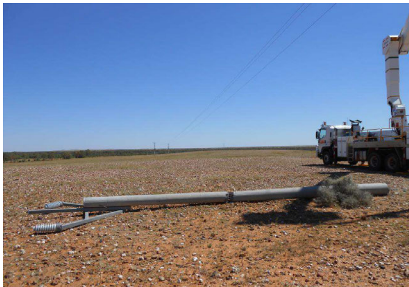
Figure 5 - Concrete Pole Failure INCD-50524-g
