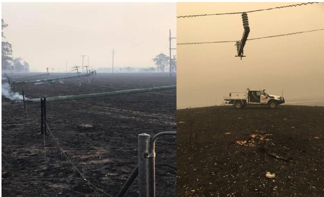
Figure 6 - Timber CCA poles 2019/20 bushfires. Right: Only a composite cross arm remaining
