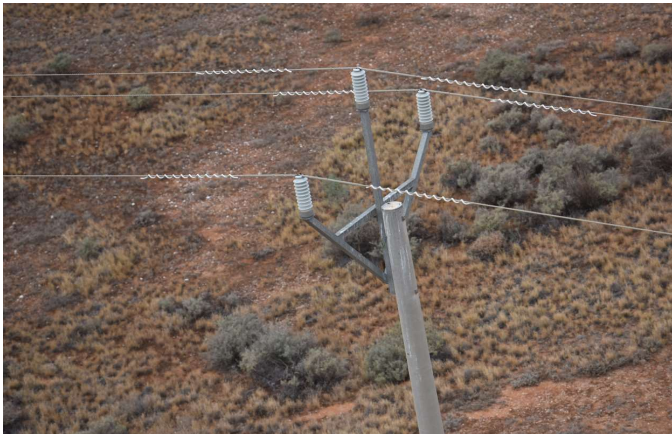
Figure 2 - Typical Pole Top Configuration
