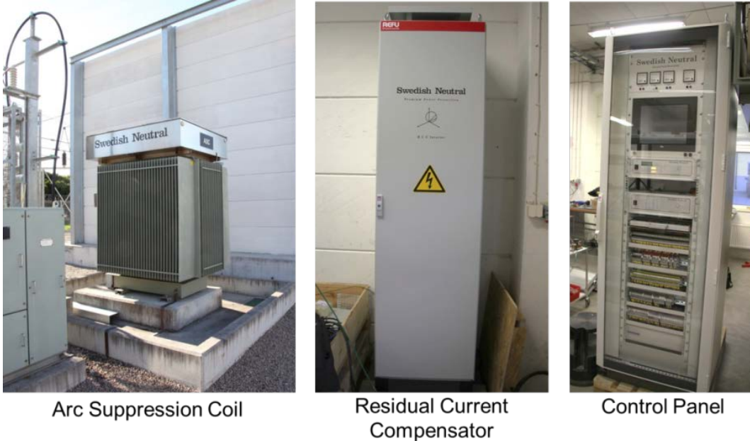
Figure 3 Components of a REFCL
