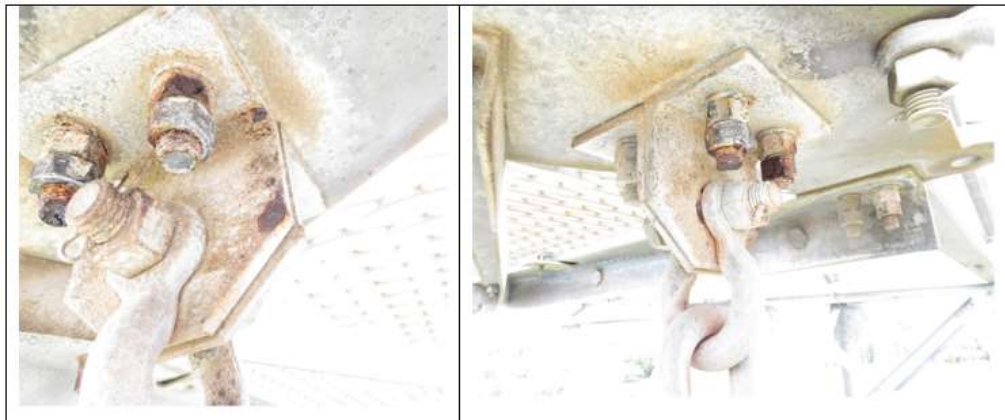
Figure 15: A small number of towers will need maintenance as in example of tower STR - 0163 (2019)
