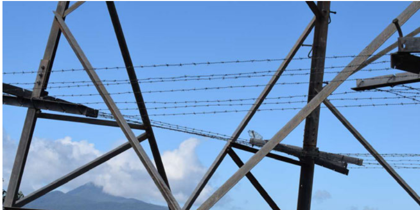
Figure 7: Climbing devices replaced - example STR - 1549 (2019)
