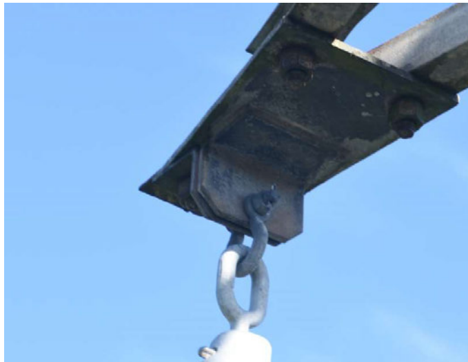
Figure 23: STR-1540 – Cold end hardware in good corrosion (2018)
