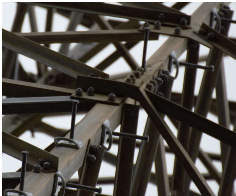
Figure 5: Typical corrosion free climbing aids - example STR - 1528 (2019)
