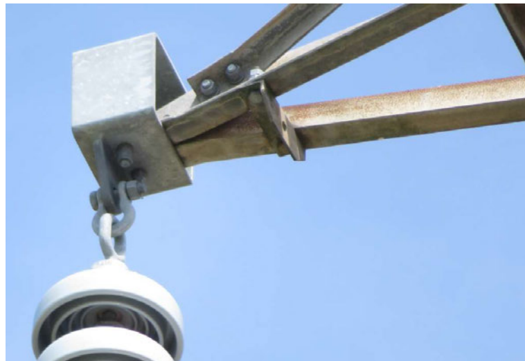
Figure 14: Replaced components in the conductor attachment area of suspension tower STR - 1544 (2019)
