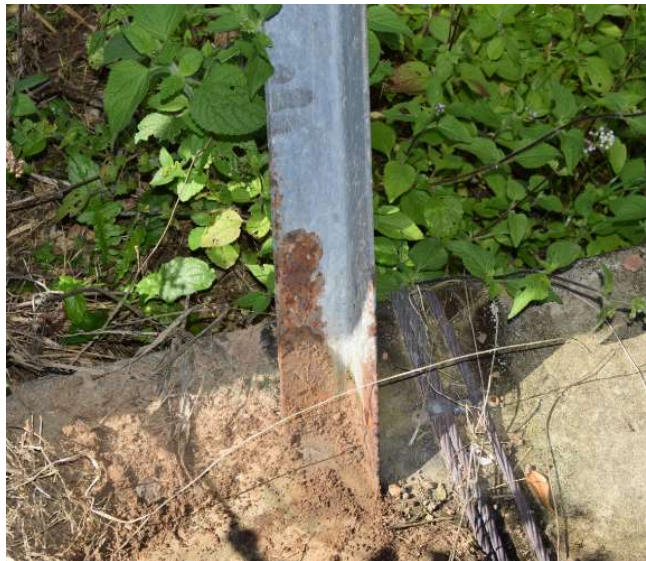
Figure 4: 1252-STR-1557 TOWER LEG (2019)
