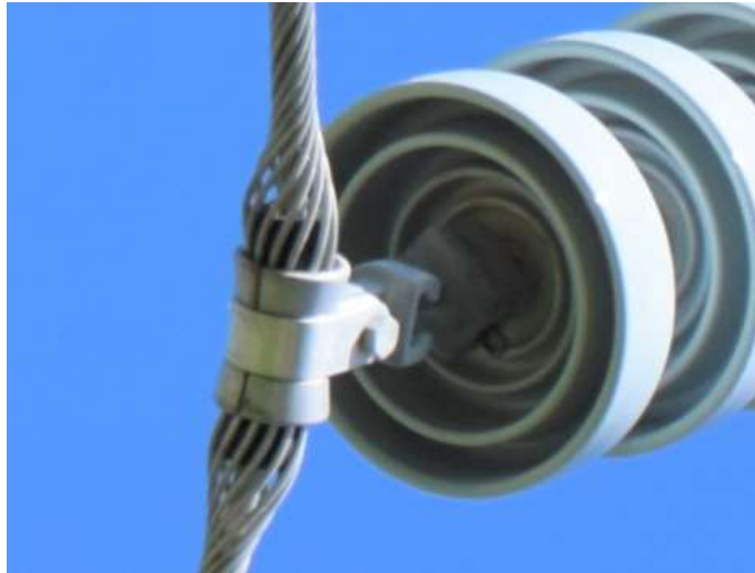
Figure 24: STR-1551 – Cold end hardware in good corrosion (2019)
