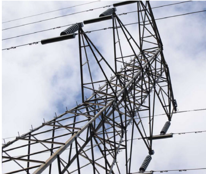
Figure 21: STR-1553 Example of dampers in good condition shown (2019)
