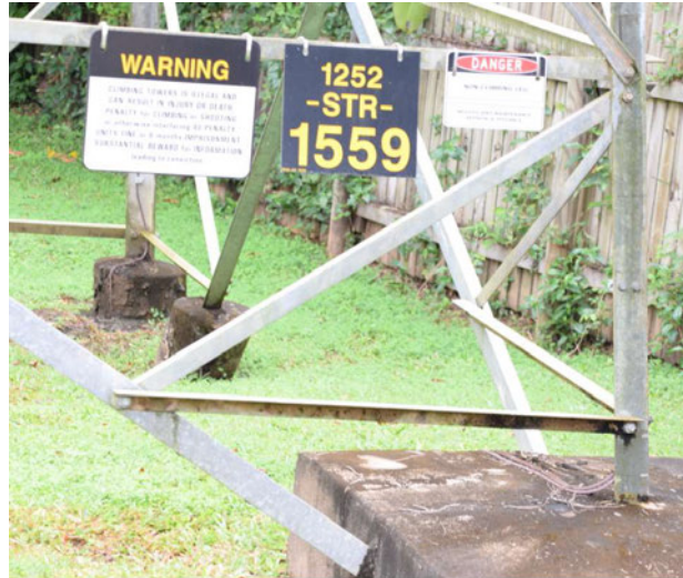
Figure 3: 1252-STR-1559 TOWER LEGS (2019)
