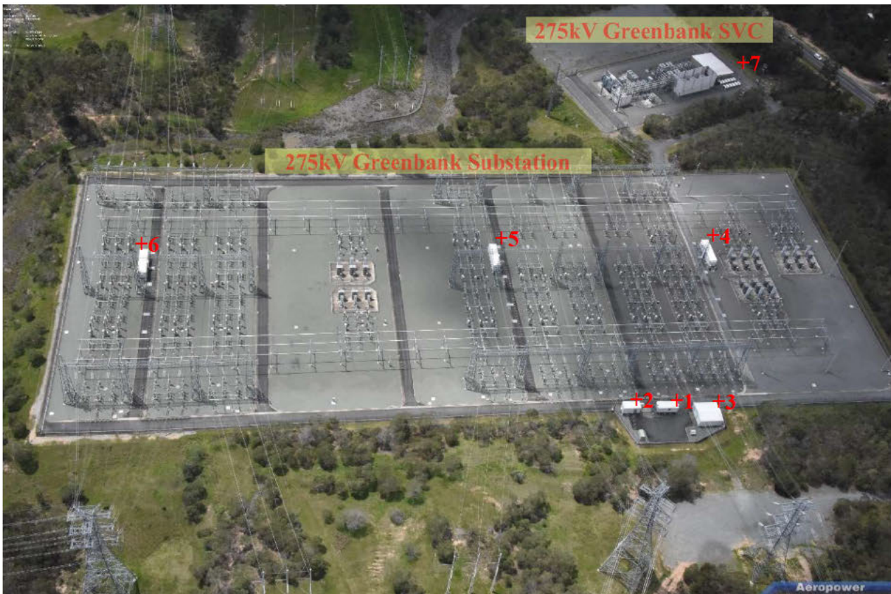
Figure 2 – 275kV Greenbank Substation Aerial View
