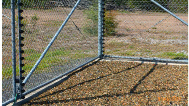
Figure 32: Asphalt along part of the outside
