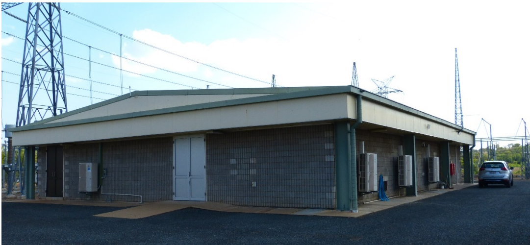
Figure 5: Control Room Building
