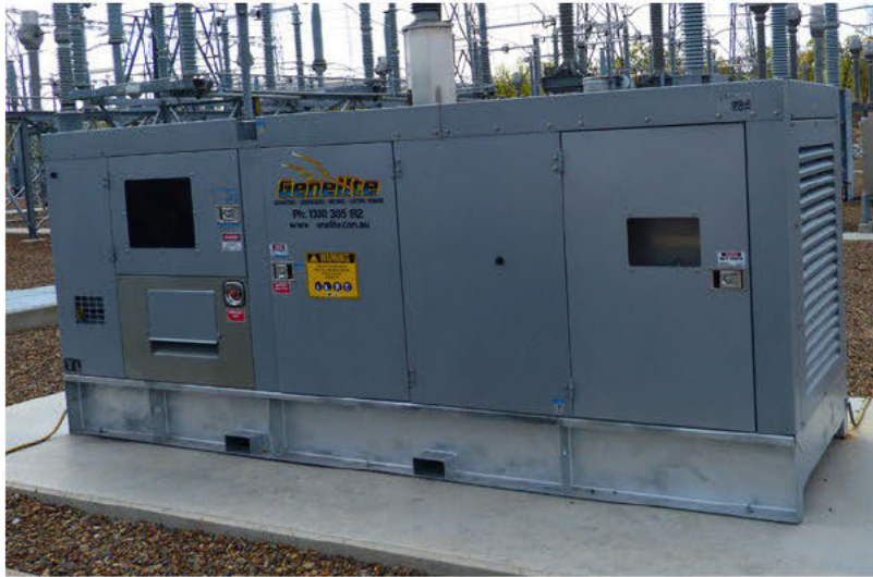
Figure 25: Diesel generator
