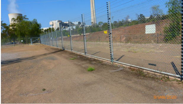
Figure 31: Gravel in the yard
