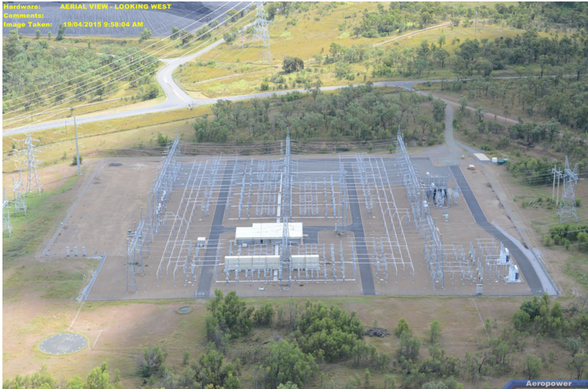
Figure 2: Aerial Photograph of H024 Calvale Substation –2015
