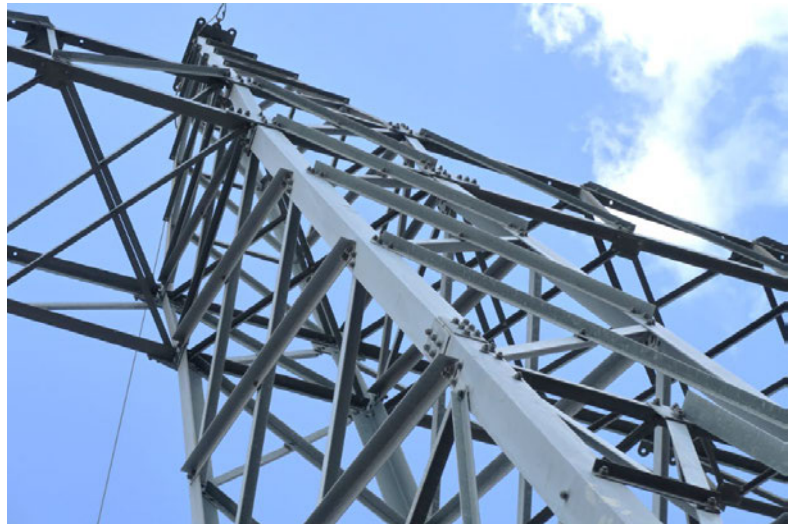
Figure 22: 275kV Structure Main Leg
