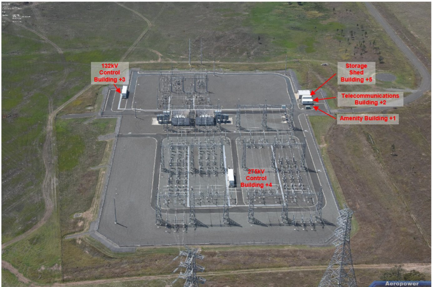
Figure 2 – 275 kV / 132kV Teebar Creek Substation Aerial View
