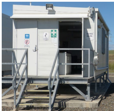
(a) Amenity Building +1 and Minor OpsWAN Equipment
