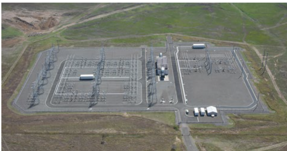
Figure 2 – H063 Teebar Creek – Aerial View looking North
