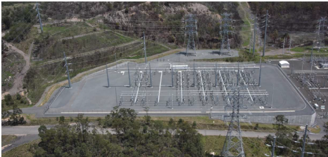
Figure 3 H072 Aerial Photo
