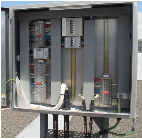
1 Transformer LV bay AC supply and VT box
