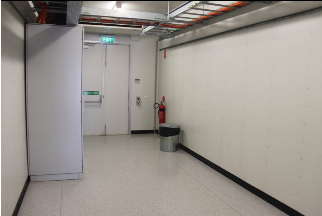
Control building +4 inside
