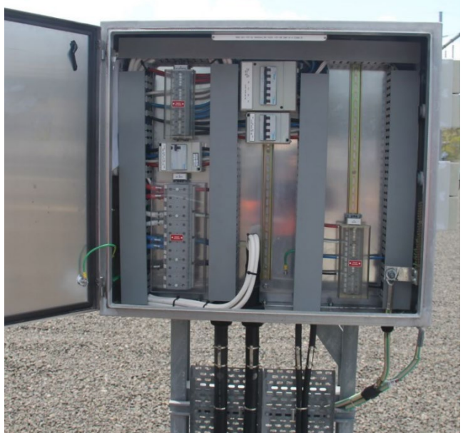
4T and 5T 110kV AC supply marshalling kiosk
