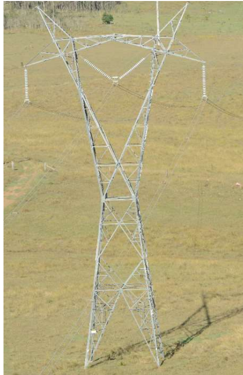
Figure 2: 1122-STR-4712 - Suspension Tower
