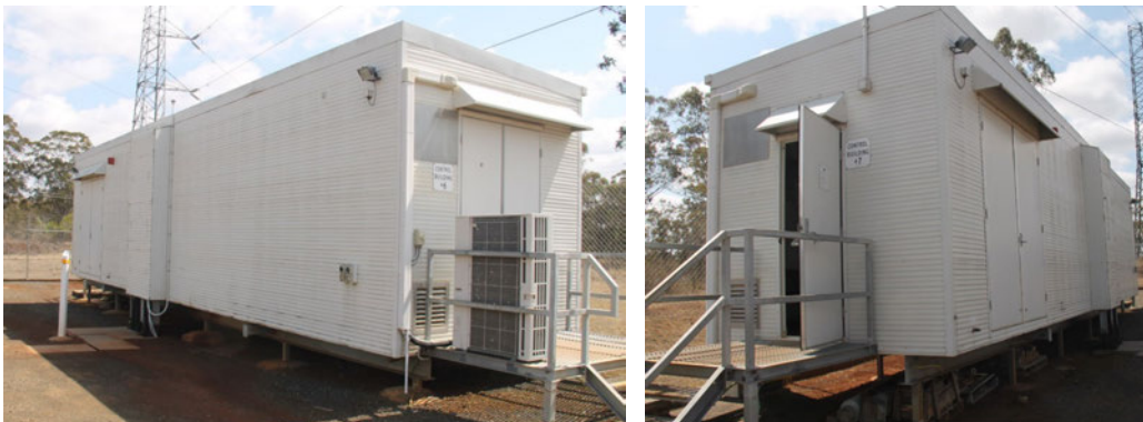
Demountable control building +6 and +7
