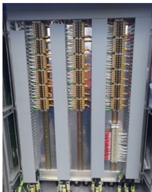
=C3.1 Feeder 8848 CB marshalling kiosk and CVT box
