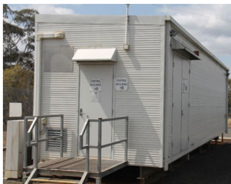
Demountable control building +8
