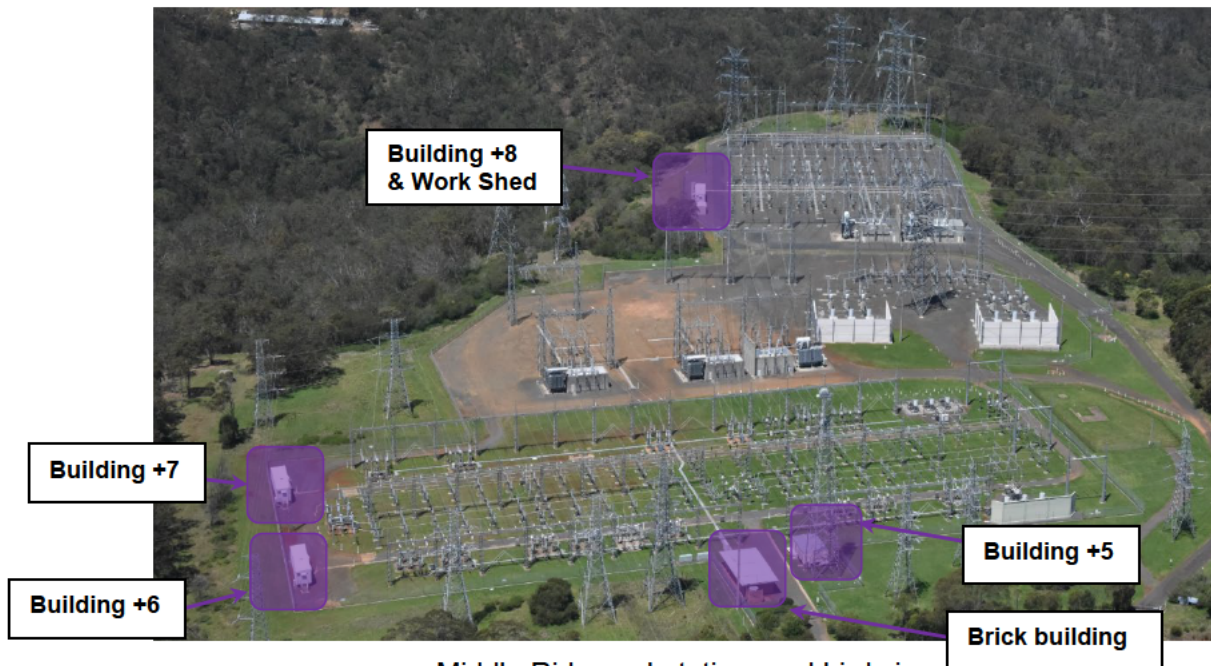
Middle Ridge substation yard bird view
