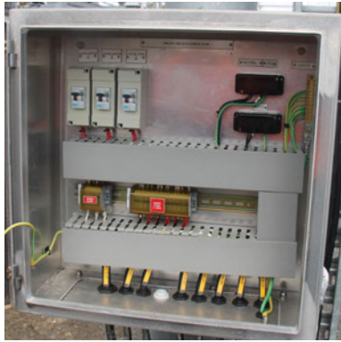
=C1 275kV Transformer 2 stub CVT box AC supply termination cubicle
