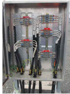
=C1 275kV Transformer 2 stub CVT box AC supply termination cubicle
