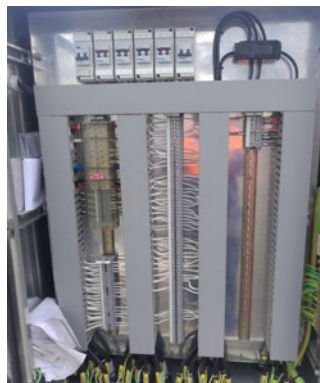
=C3.1 Feeder 8848 CB marshalling kiosk and CVT box
