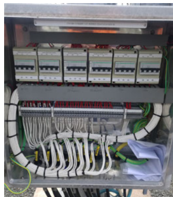
=C3.1 Feeder 8848 CB marshalling kiosk and CVT box
