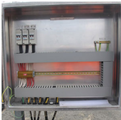
=C3 275kV AC and DC marshalling kiosk
