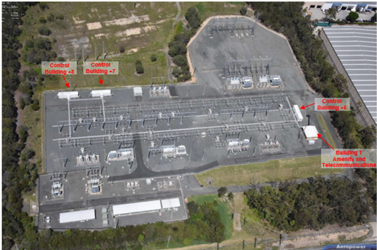
Figure 1 – 275 kV / 110kV Molendinar Substation Aerial View
