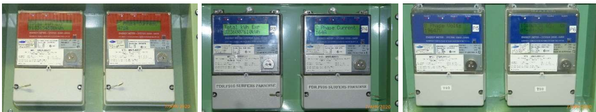
Figure 10 – Molendinar substation typical revenue meters
