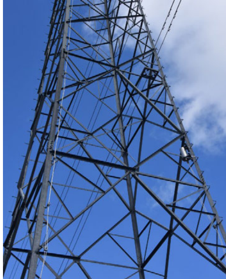
Figure 11: STR-0050 Tower body in good condition (2018)
