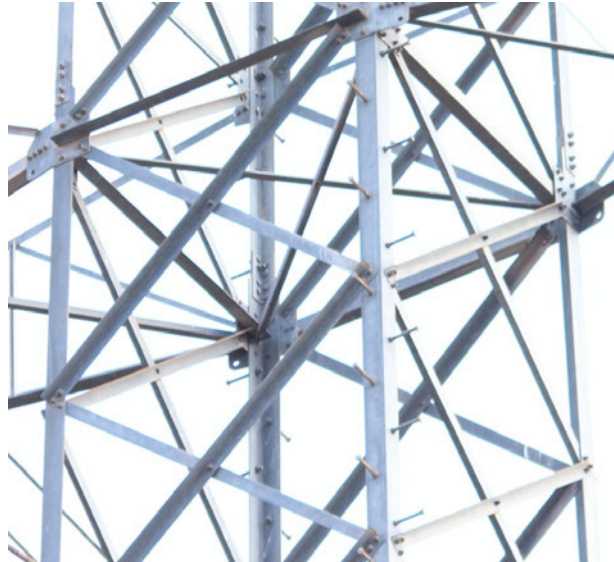
Figure 13: STR-0021 with G3 bolts and G2 on members (2018)
