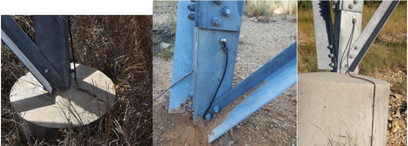
Figure 21: BS1235 Examples earthing (2016)
