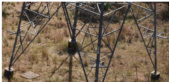
Figure 8: STR-0045; ACB barbed wire typical for towers on the line (2018)
