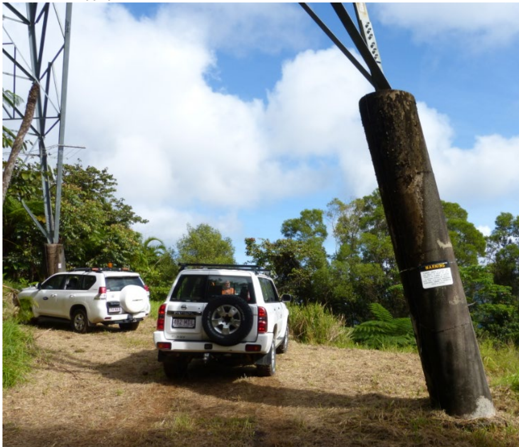
Figure 4: Extended columns on Structure 0116
