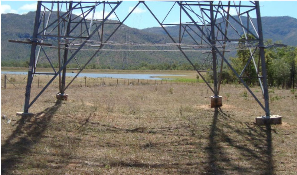
Figure 5: 1235-STR-0002 typical interface condition on the line (2015)
