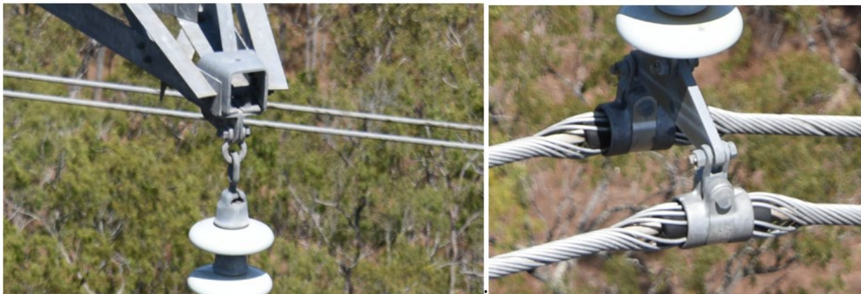
Figure 28: STR-0080 – Hardware in good condition (2018)
