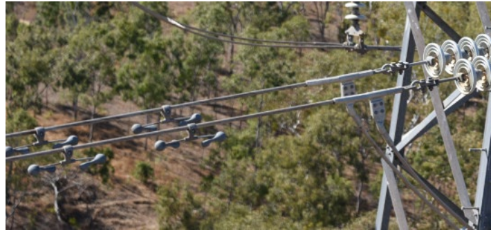
Figure 22: STR-0020 Vibration Dampers and Dead Ends (2018)
