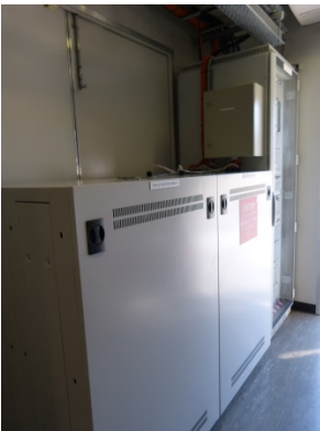
Building +C - 125VDC Batteries and Chargers
