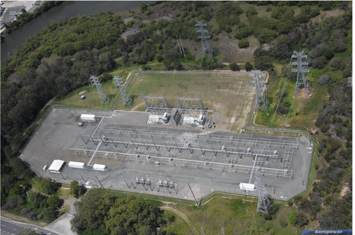
Figure 1 - H021 Murarrie 275/110kV Substation Aerial View
