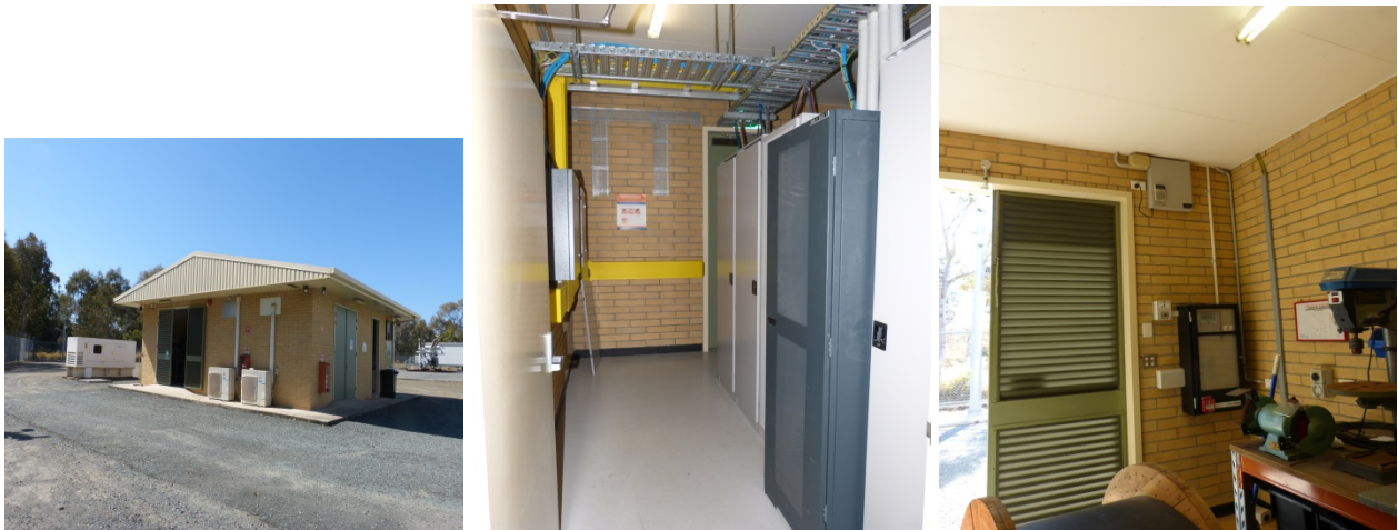
Figure 2 - H021 Murarrie Brick Building “+T”
