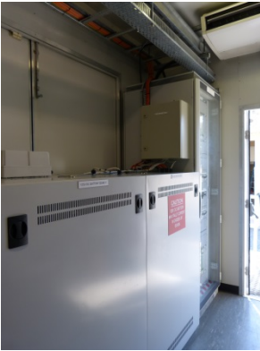
Building +A – 125VDC Batteries and Chargers
