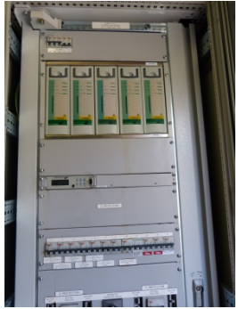
Building +B – 125VDC Batteries and Chargers
