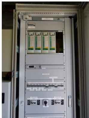
Building +C - 125VDC Batteries and Chargers
