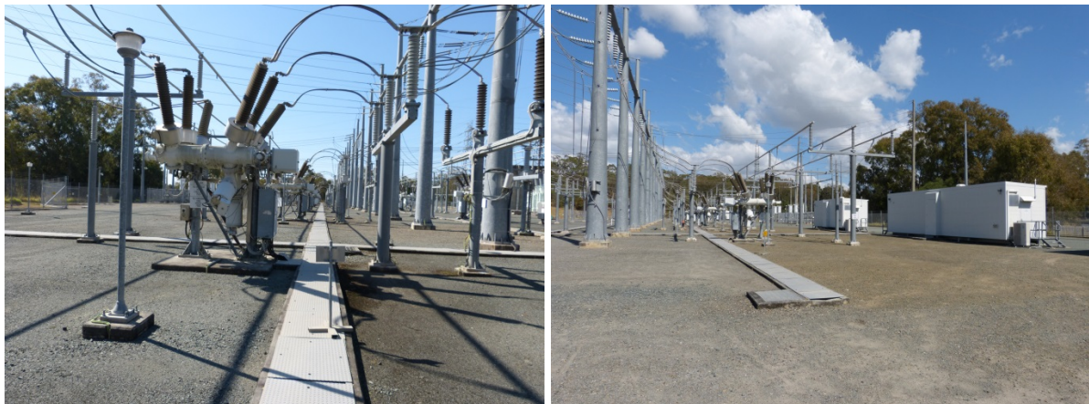
Figure 7 - Murarrie 110kV Cable Trenches
