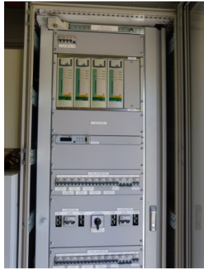
Building +A – 125VDC Batteries and Chargers
