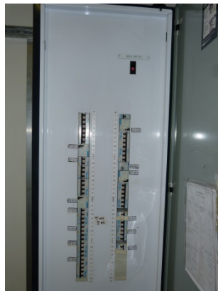
110kV building +A
