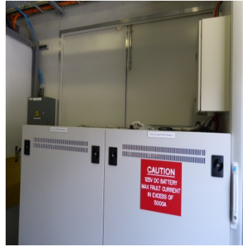
Building +B – 125VDC Batteries and Chargers
