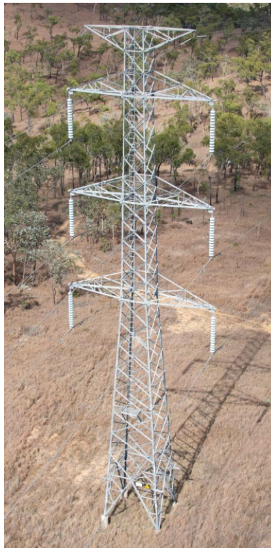
Figure 5: 1220-STR-7896 - Suspension Tower
