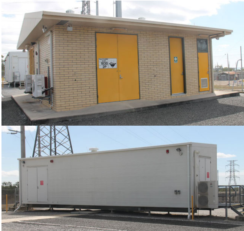
T152 Sub building T and K
