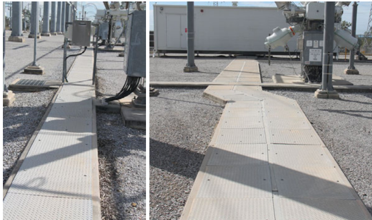
Trenches at T152
