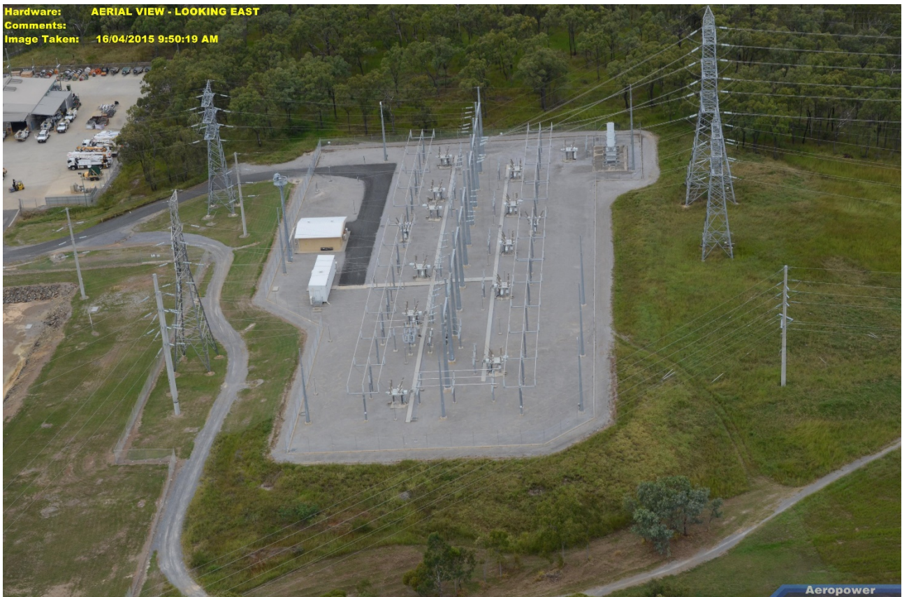
T152 Gladstone South Substation
