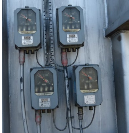
Figure 45 - HV WTI instrument, LV WTI instrument and OTI instrument. All the viewing windows are clear enabling easy instrument reading except the OTI
