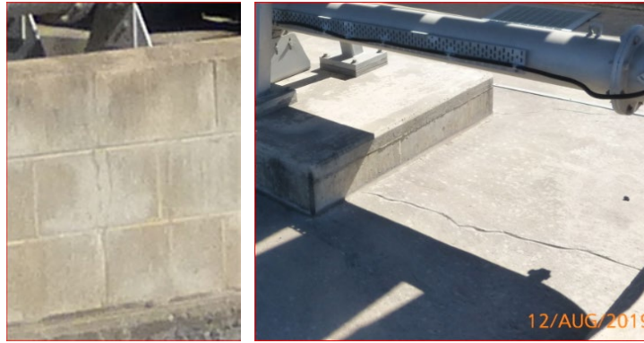
Figure 54-Bund cracks
