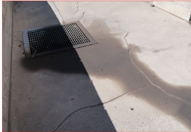
Figure 23 – Sealed cracks in bund floor
