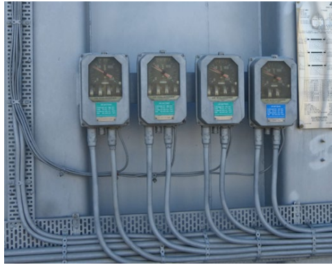
Figure 13 - HV WTI instrument, LV WTI instrument and OTI instrument. All the viewing windows are clear enabling easy instrument reading except the OTI.
