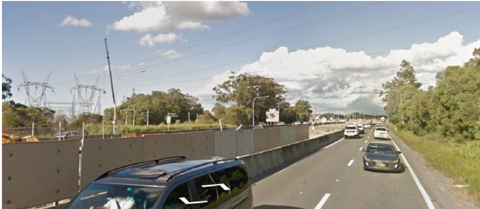
Figure 12: BS1018 and 1019 M1 Motorway crossing near Mudgeeraba Substation
