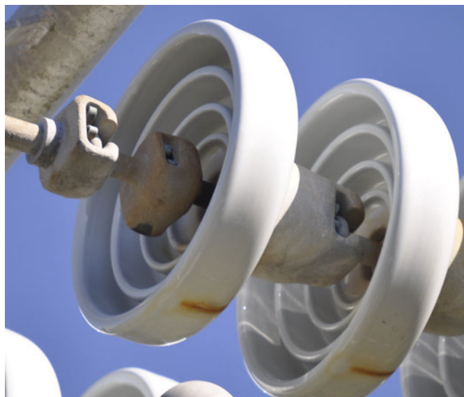
Figure 27: 1019-STR-3372 Tension String
