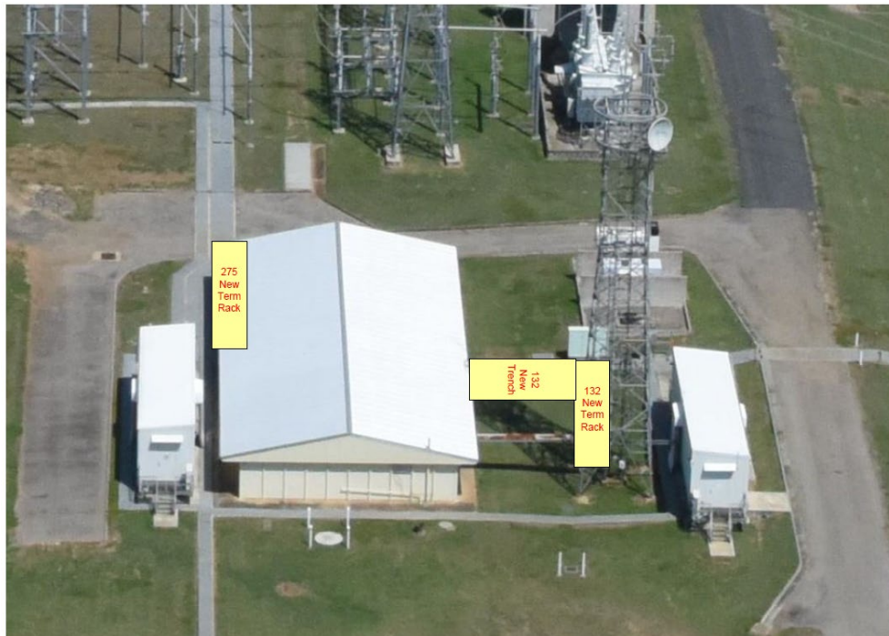
Figure 3-3: 132kV/275kV Woolooga Substation proposed termination rack locations
