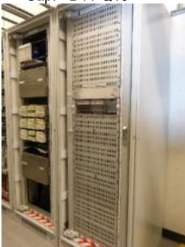
Power Quality Monitoring
