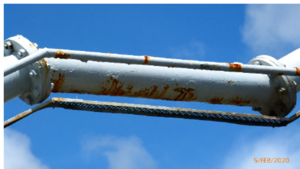
Figure 4: Corrosion on the conservator pipe work and on the base plate of A
