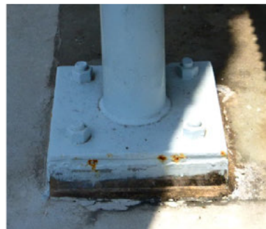
Figure 3: Grade 4 corrosion on the base plate of the transformer
