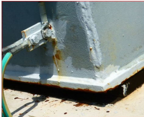
Figure 18- Corrosion in 2020
