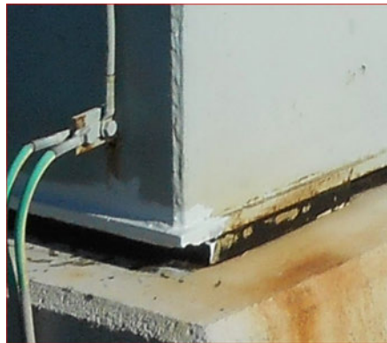
Figure 19 – Corrosion in 2015
