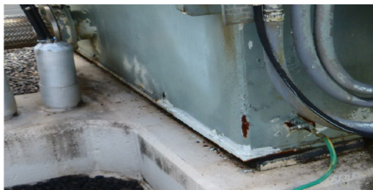
Figure 3: Grade 4 corrosion on the base plate of the transformer
