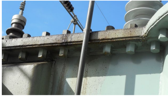
Figure 4 Welded steel strap between main tank and lid, complete with 'O'-ring sealed dome nuts
