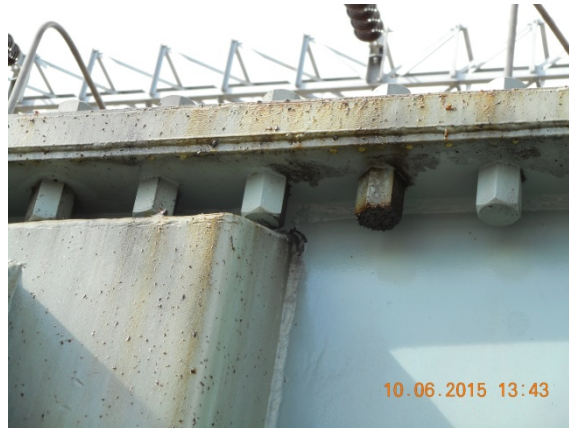
Figure 27 Welded steel strap between main tank and lid, complete with 'O'-ring sealed dome nuts.
