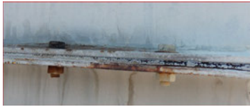
Figure 7 –Corrosion Grade 2
