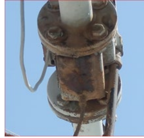
Figure 6 – Grade 3 Corrosion
