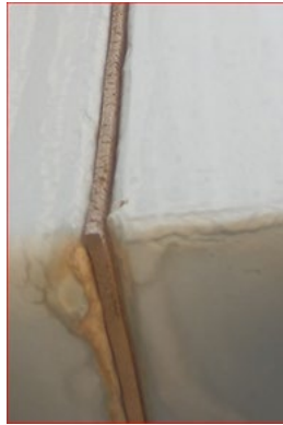
Figure 14 – Deteriorated Gasket
