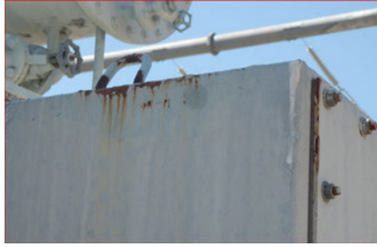
Figure 5 - Grade 2 Corrosion
