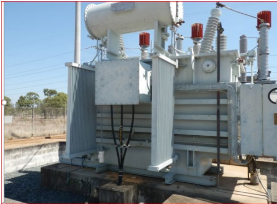
Figure 27 – 11 kV Cable Air Termination Box
