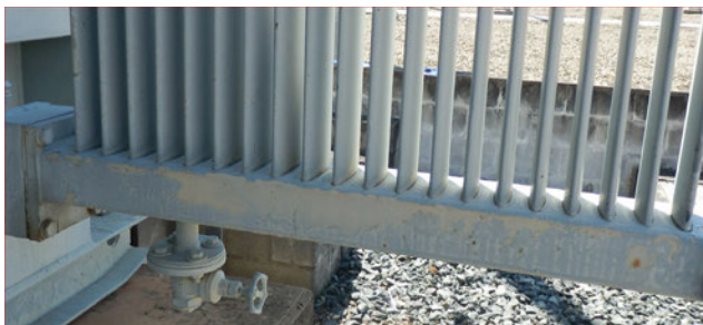
Figure 30 – Peeling paint
