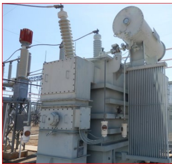
Figure 15 – Three desiccant breathers
