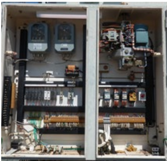
Figure 16 – WTI and OTI (Installed in Shared Control Cubicle)
