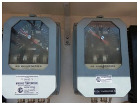
Figure 16 – WTI and OTI (Installed in Shared Control Cubicle)
