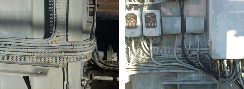
Figure 37: The painted multicore cables are looking aged but still serviceable.
