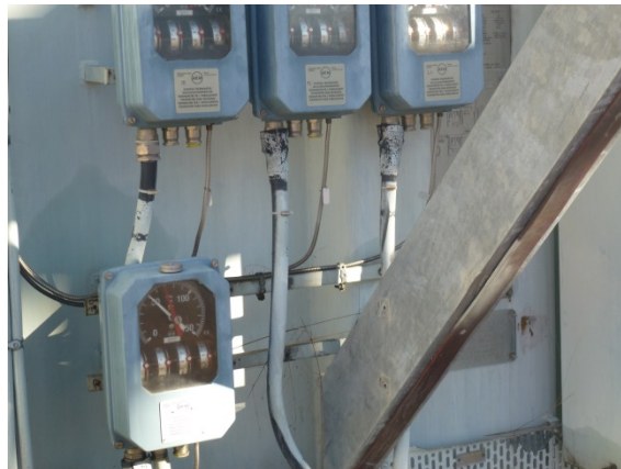
Figure 26: Kihlstrom temperature measurement instrumentation appears to be in good condition following some replacements in later years.
