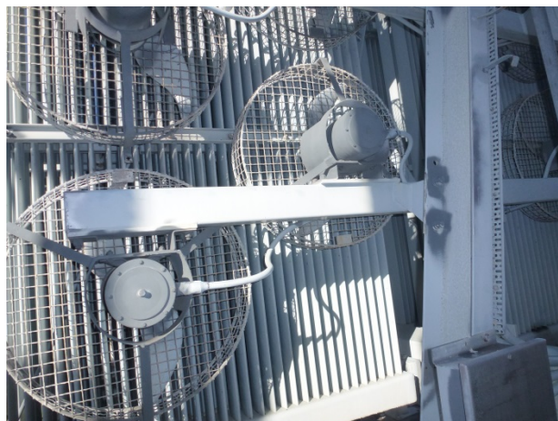
Figure 18: Cold galvanising paint applied to fan body, casings and mounting brackets.
