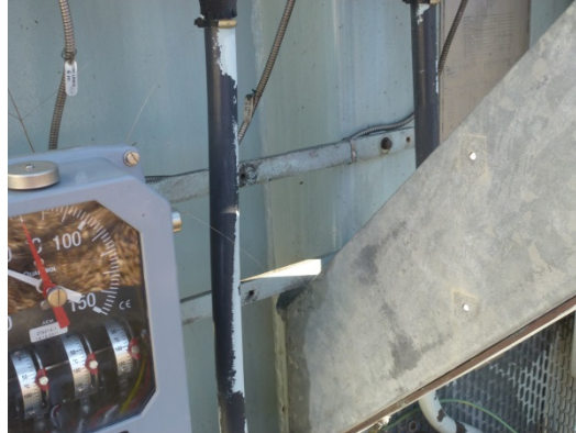
Figure 12: Kihlstrom temperature measurement instrumentation appears to be in good condition following replacement in later years.
