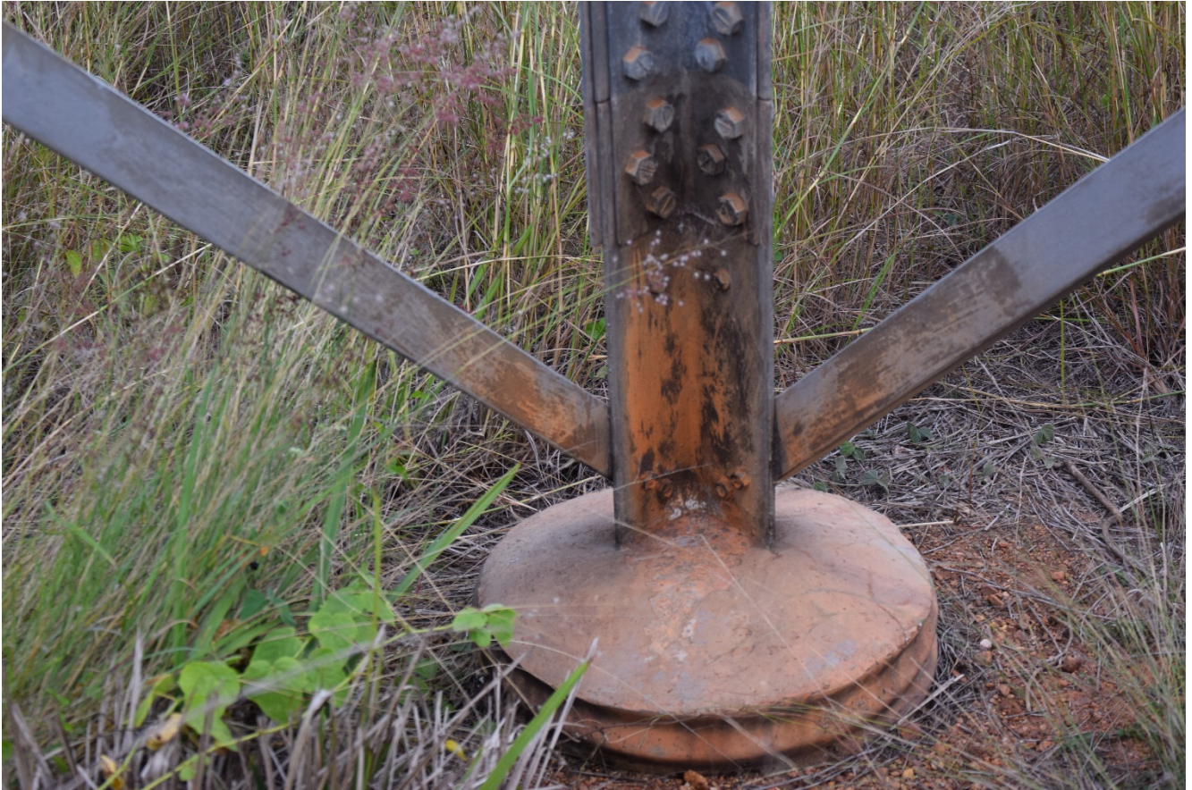
Figure 3: 1515-STR-0019 Tower Leg Condition
