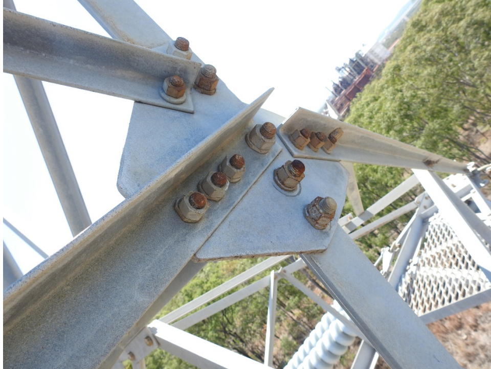
Figure 9: 1515-STR-0017 with G2 and G3 bolts
