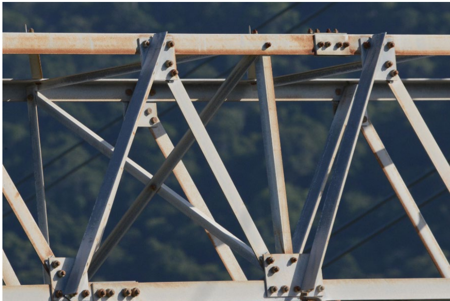
Figure 10: 1515-STR-0028 Superstructure G3 bolts and G2 members
