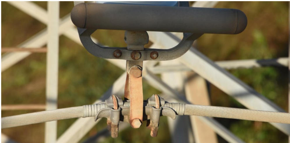
Figure 30: 1515-STR-0012 Bridging Insulator Hardware - Hot End
