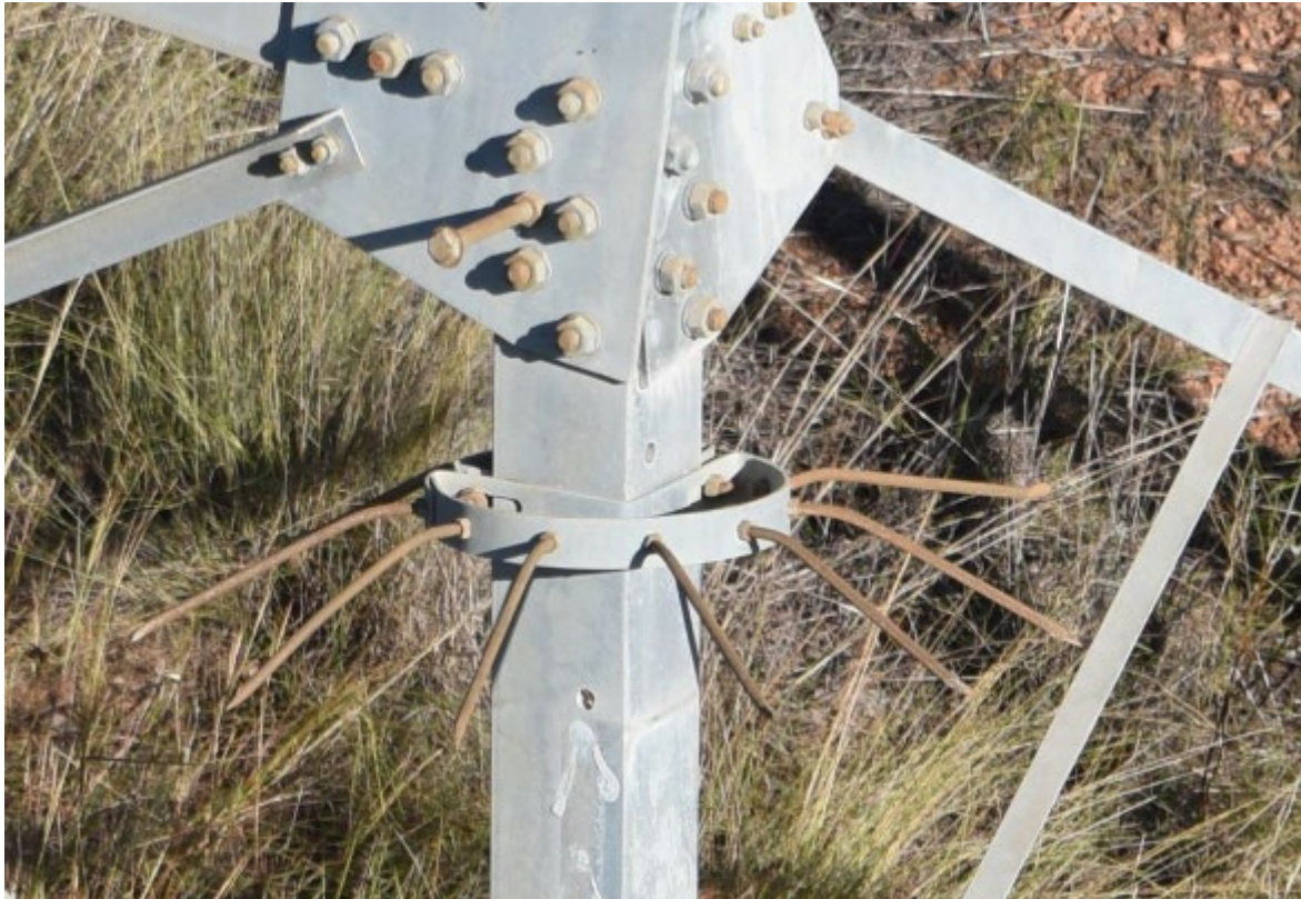
Figure 6: 1515-STR-0017 ACB Crown of Thorns
