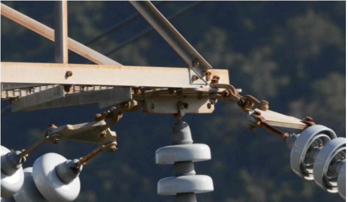
Figure 28: 1515-STR-0028 Tension Tower Attachment Location
