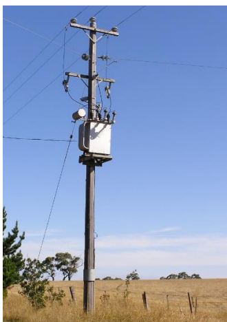
Figure A1-4: Picture of a typical pole mounted distribution substation
