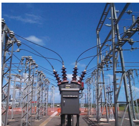
Figure A1-5: Picture of a Circuit Breaker within a Zone Substation
