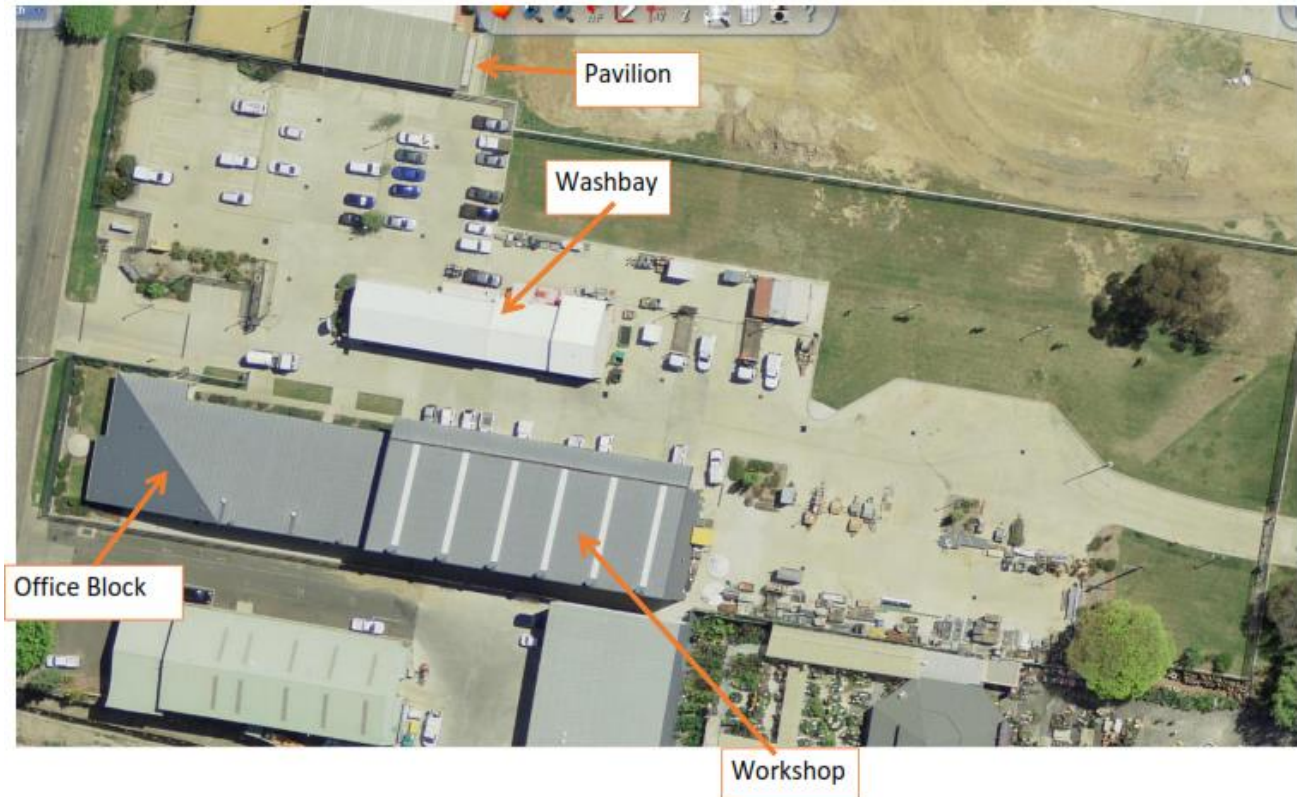
Orange Depot – Image courtesy of Google Earth
