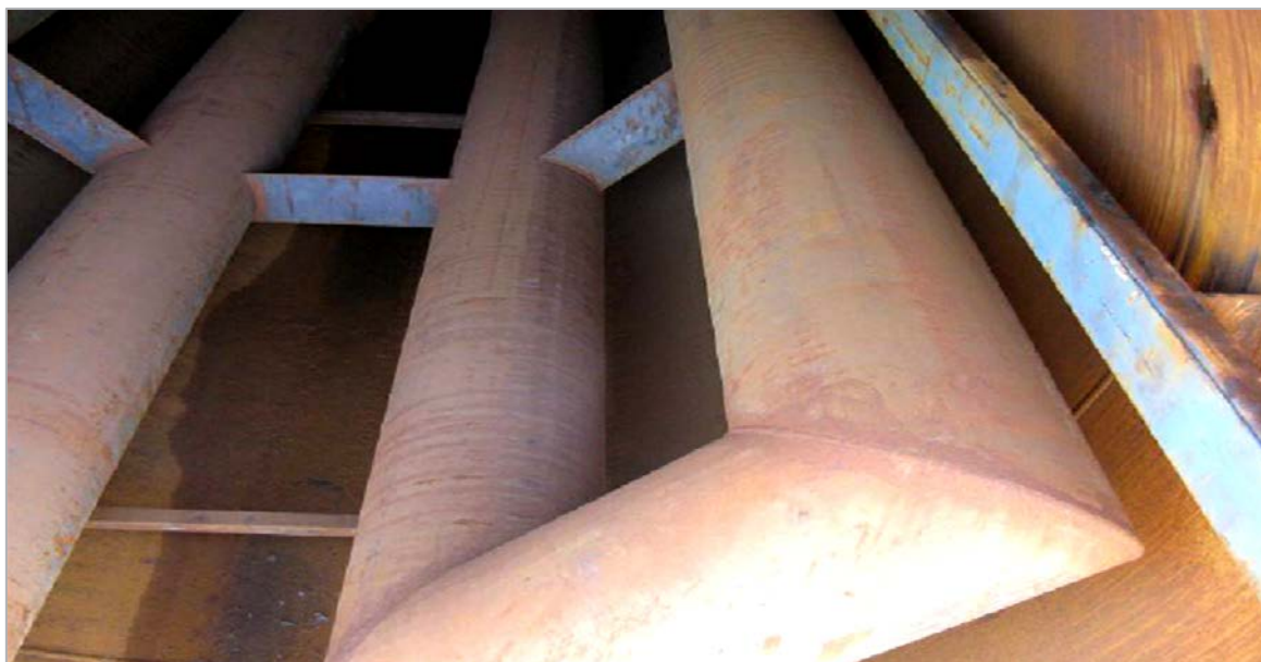
Figure 2-4: Fire tubes of a Water Bath Heater
