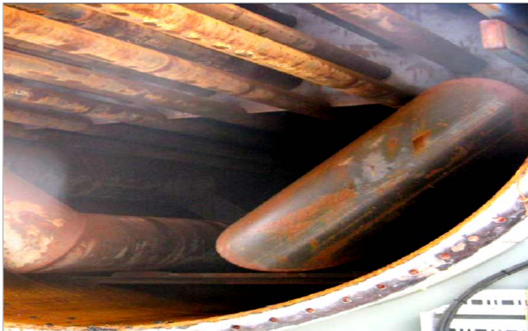
Figure 2-5: End view of a Water Bath Heater
