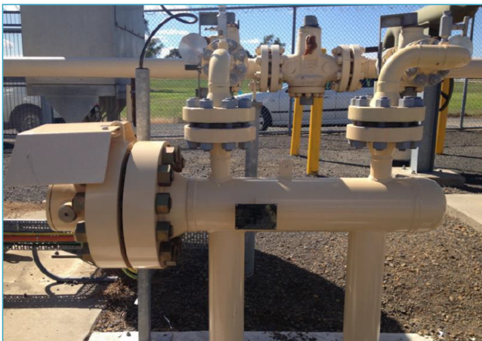
Figure 3-7: [REDACTED] city gate electric gas heater
