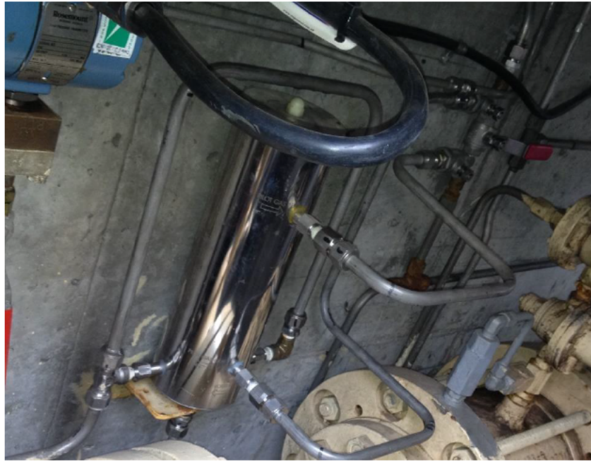
Figure 3-8: Vortex Heater Installation
