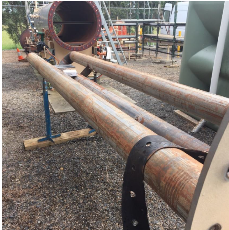
Figure 3-5: End view of a water bath heater
