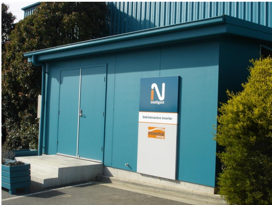
Figure 1 Queanbeyan Inverter Installation
