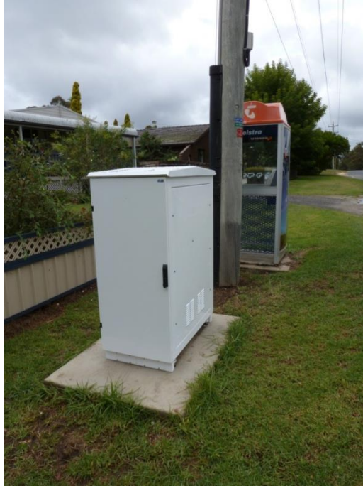
Figure 3 Bega / Kalaru Inverter Installation
