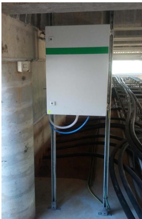
Clearwater Zone Substation 5kVA four quadrant inverter (atypical) installation
