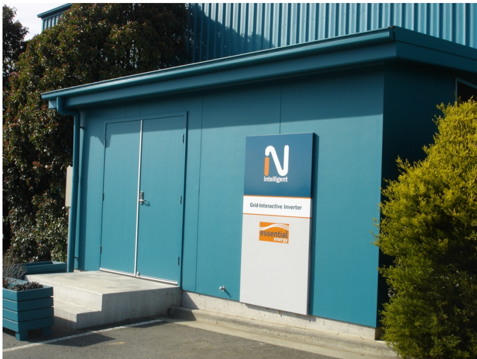
Figure 1 Queanbeyan Inverter Installation
