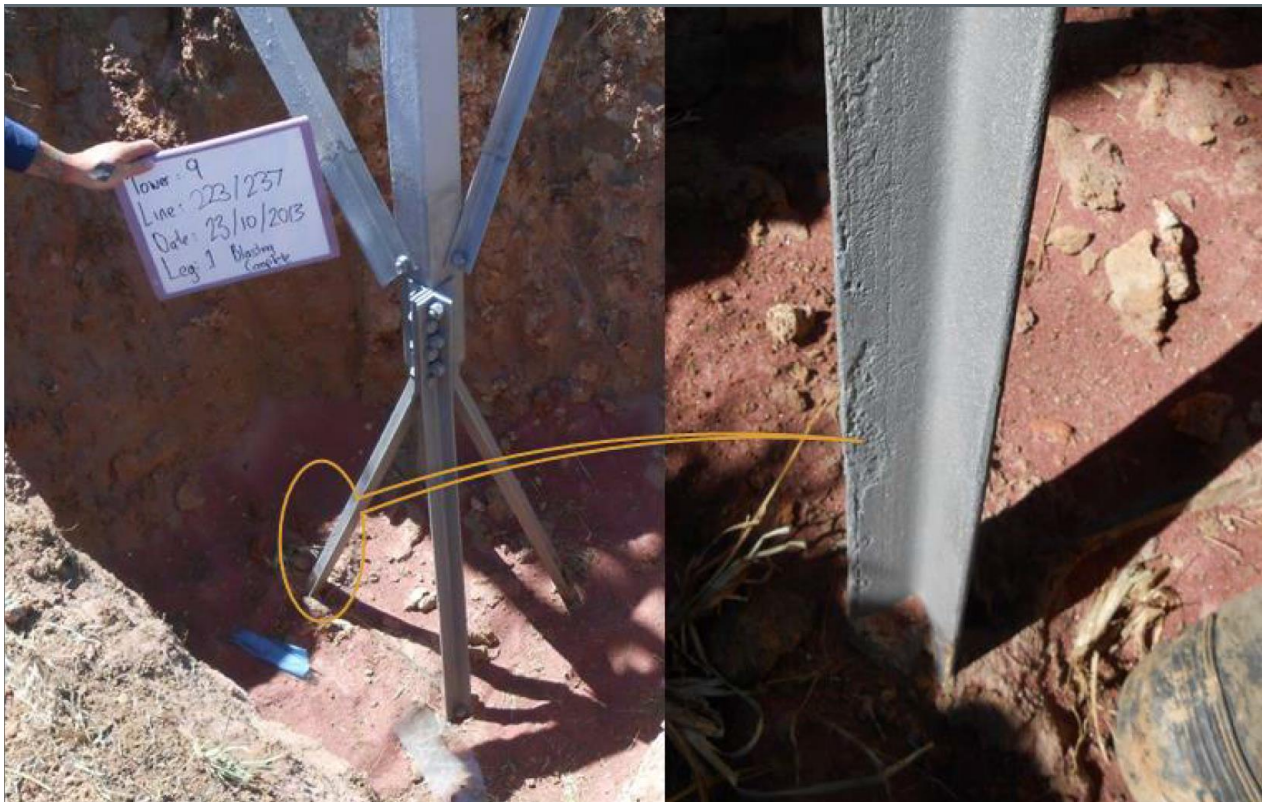
Grillage foundation with minor corrosion damage, after refurbishment.
