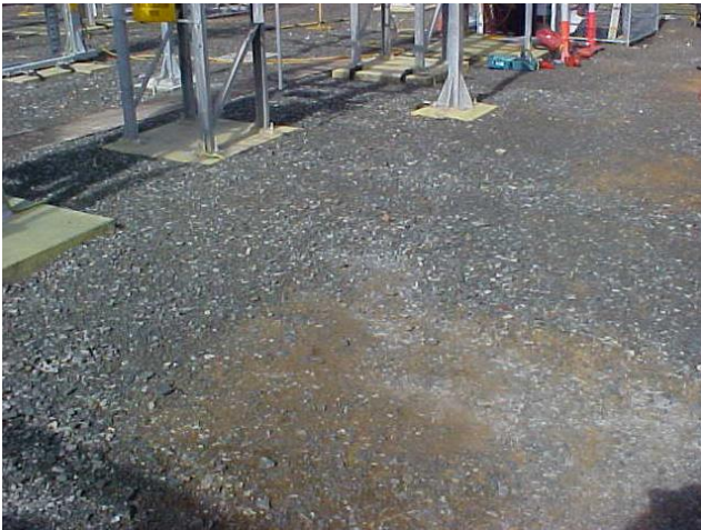
Figure 3: Smithfield ZS switchyard gravel depth < 20mm
